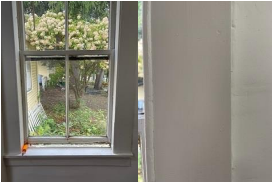
Closeup Restored Interior Frames (all original wood)
