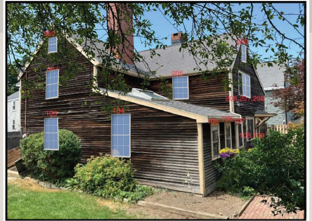
#302 Double-Hung (DG), Reverse Cottage 2:1, Exterior White #103, #104, #204, #207- #208 , Double-Hung (DG), 1:1, Exterior White, Glass: All Sash: High Performance SmartSun with HeatLock Glass, White, Window, Opening Control Device, Grille Style: Full Divided Light (FDL with spacer) Grille Pattern: All Sash: Colonial 2w x 2hC
