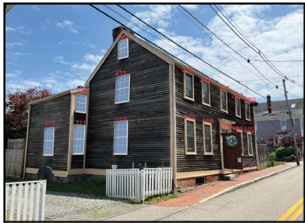
#301 Double-Hung (DG), Reverse Cottage 2:1, Exterior White #210, #211, #110, #111, #112 Double-Hung (DG), 1:1, Exterior White, Glass: All Sash: High Performance SmartSun with HeatLock Glass, White, Window, Opening Control Device, Grille Style: Full Divided Light (FDL with spacer) Grille Pattern: All Sash: Colonial 2w x 2h
