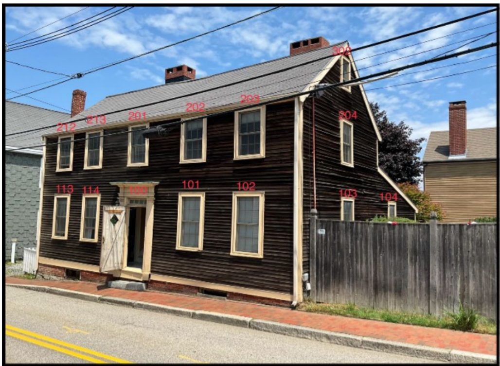
EXTERIOR – FRONT / SIDE
