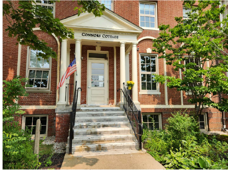
VIEW OF EXISTING SOUTH ENTRY
