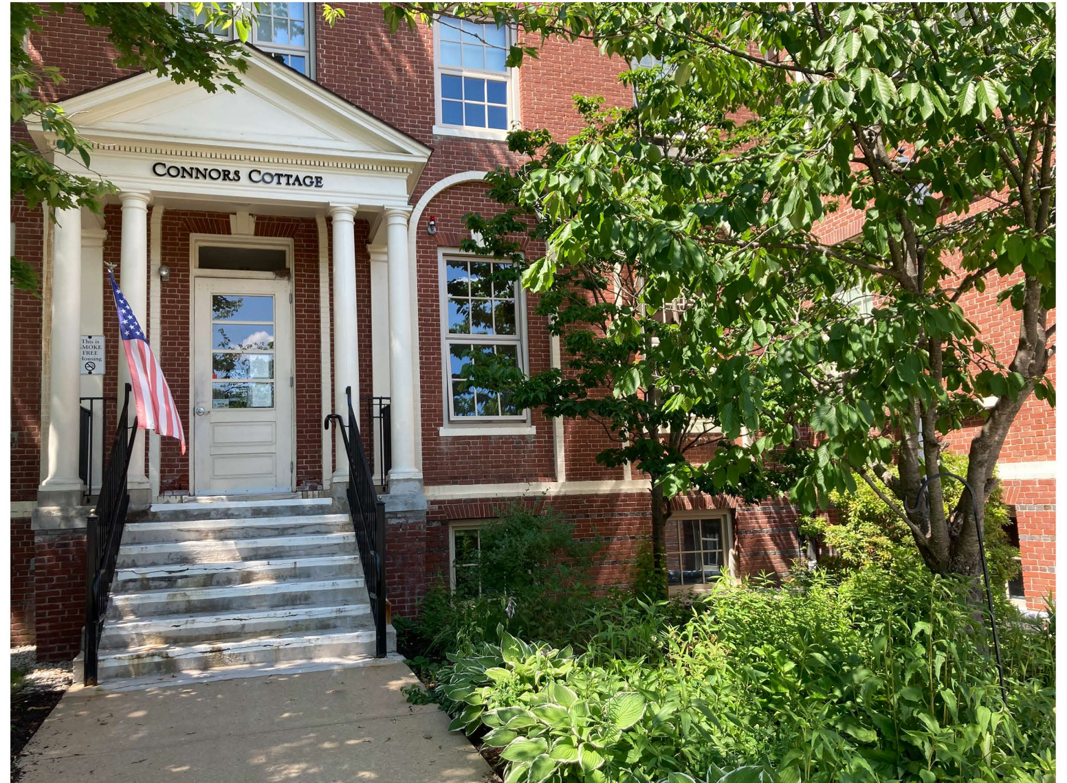
VIEW OF EXISTING SOUTH ENTRY
