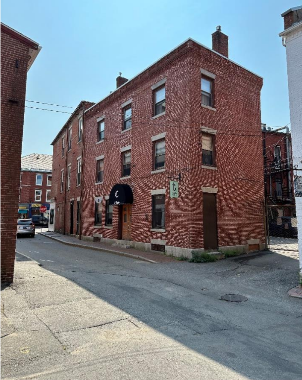
Figure 1 18 Ladd Street from South West
