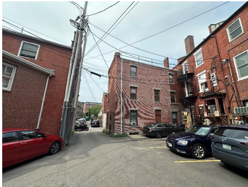
Figure 4 18 Ladd Street from Atheneum Courtyard
