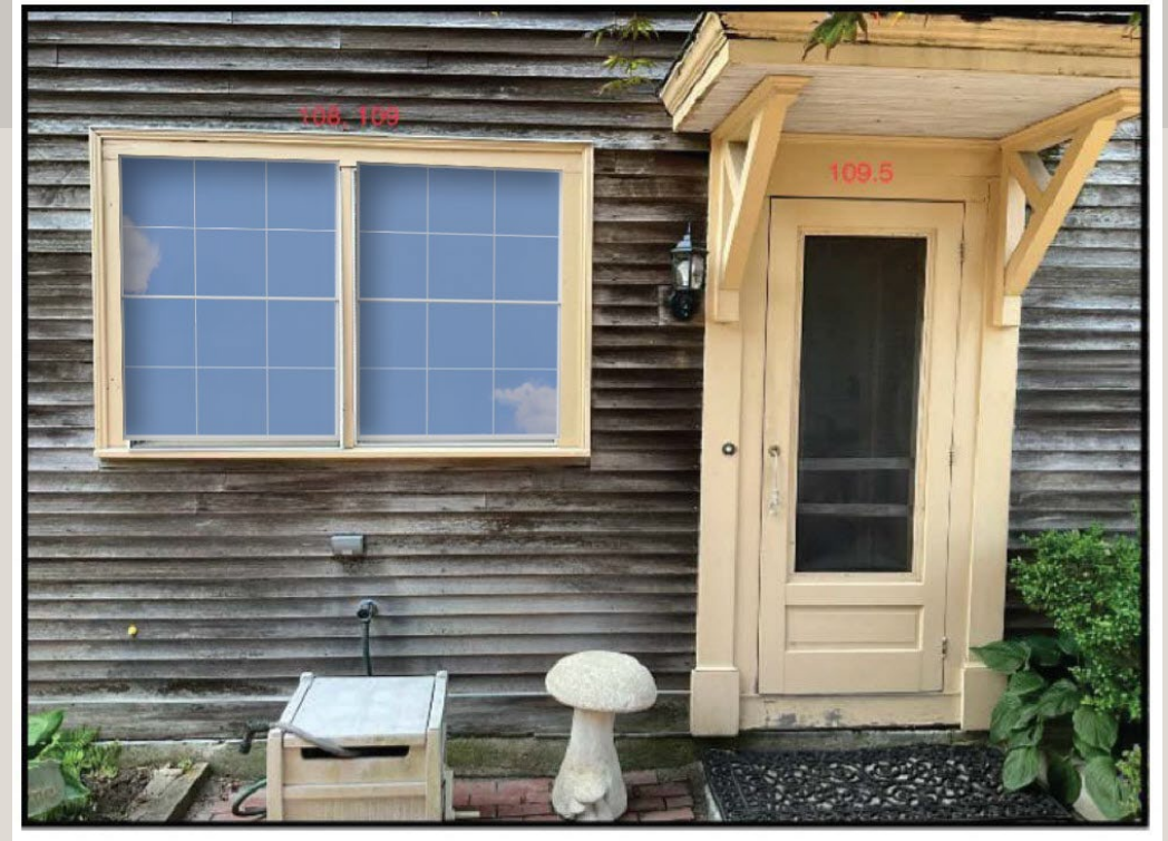
#108, #109 Double-Hung (DG), 1:1, Exterior White, Glass: All Sash: High Performance SmartSun with HeatLock Glass, White, Window, Opening Control Device, Grille Style: Full Divided Light (FDL with spacer) Grille Pattern: All Sash: Colonial 2w x 2h
