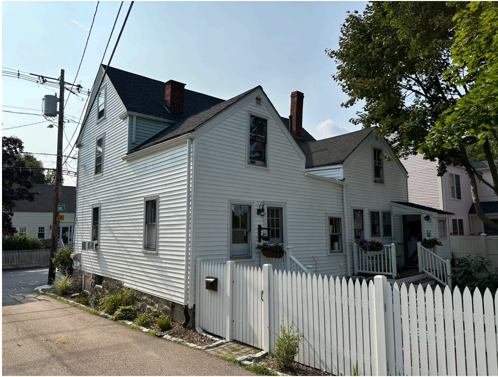
Image #5. EXISTING RIGHT AND REAR ELEVATIONS VIEW FROM HOLMES COURT, MARCY STREET AT FAR LEFT, both chimneys visible
