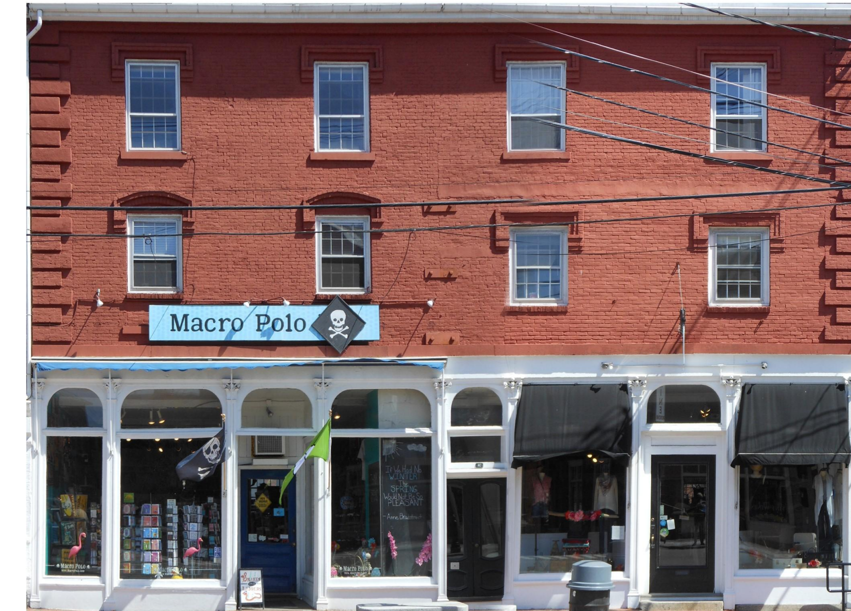
EXISTING MARKET STREET ELEVATION REFERENCE PHOTO: NOT TO SCALE
