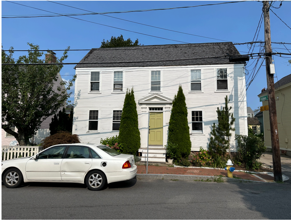
Image #3. EXISTING FRONT ELEVATION VIEW FROM MARCY STREET, no chimneys visible
