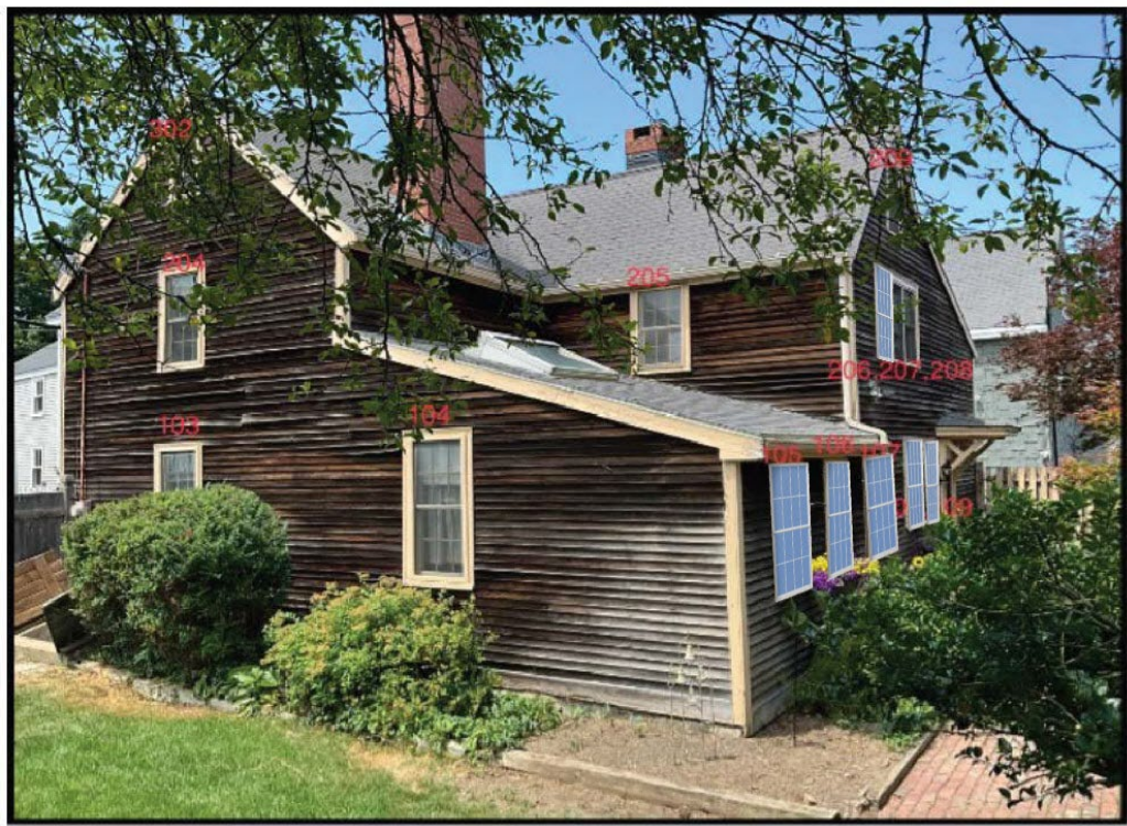
#206, #105 - #109 Double-Hung (DG), 1:1, Exterior White, Glass: All Sash: High Performance SmartSun with HeatLock Glass, White, Window, Opening Control Device, Grille Style: Full Divided Light (FDL with spacer) Grille Pattern: All Sash: Colonial 2w x 2h
