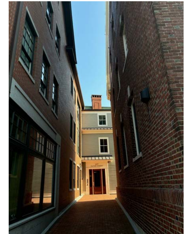
FROM DANIEL STREET LOOKING SOUTH
