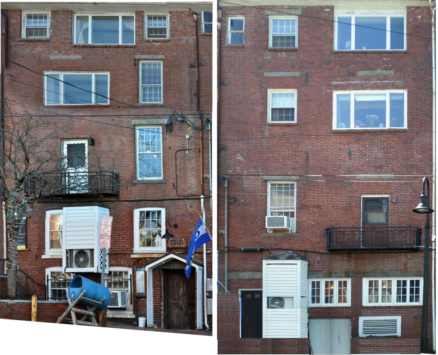
EXISTING CERES STREET ELEVATION REFERENCE PHOTO: NOT TO SCALE
