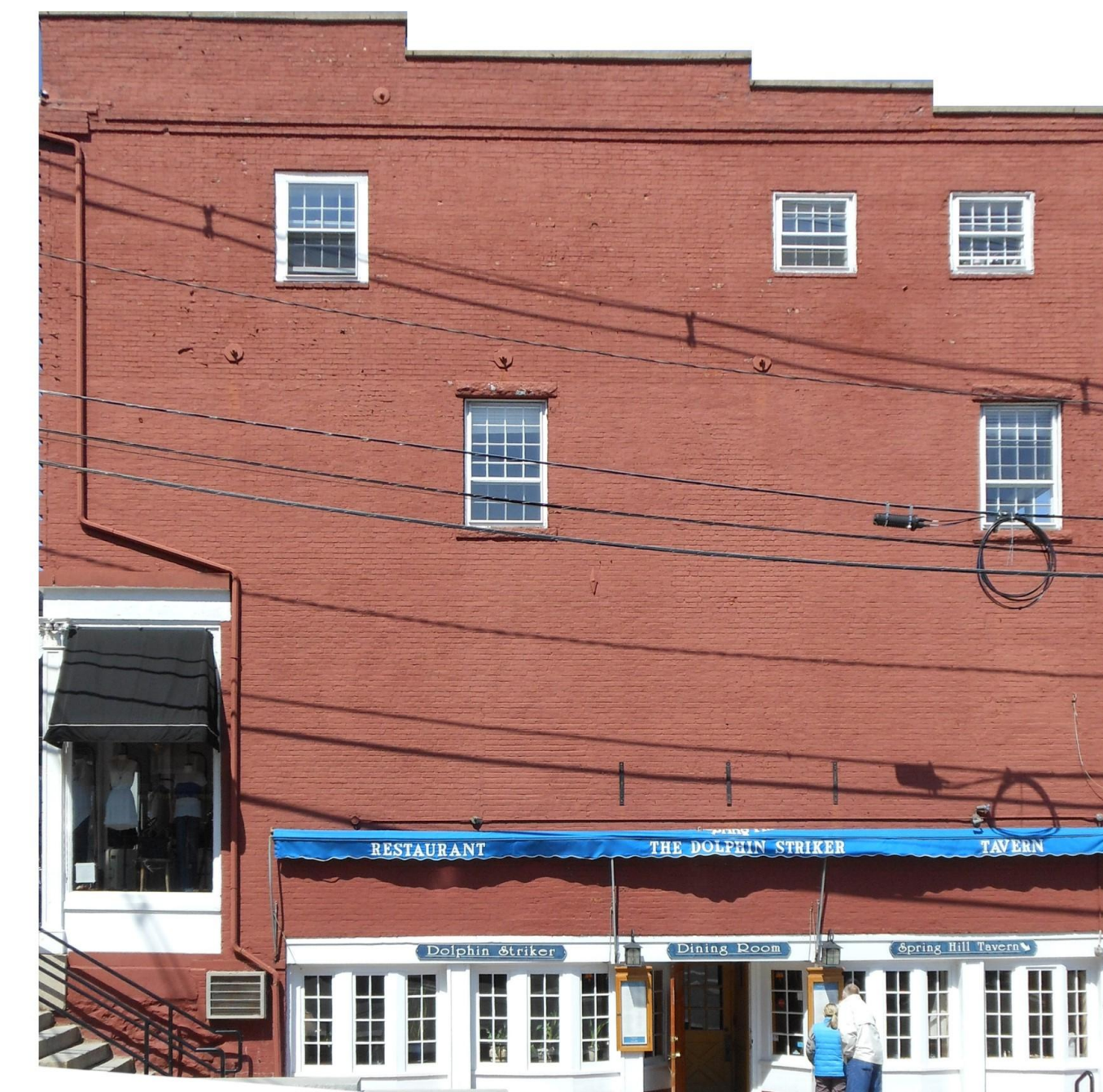
EXISTING BOW STREET ELEVATION REFERENCE PHOTO: NOT TO SCALE
