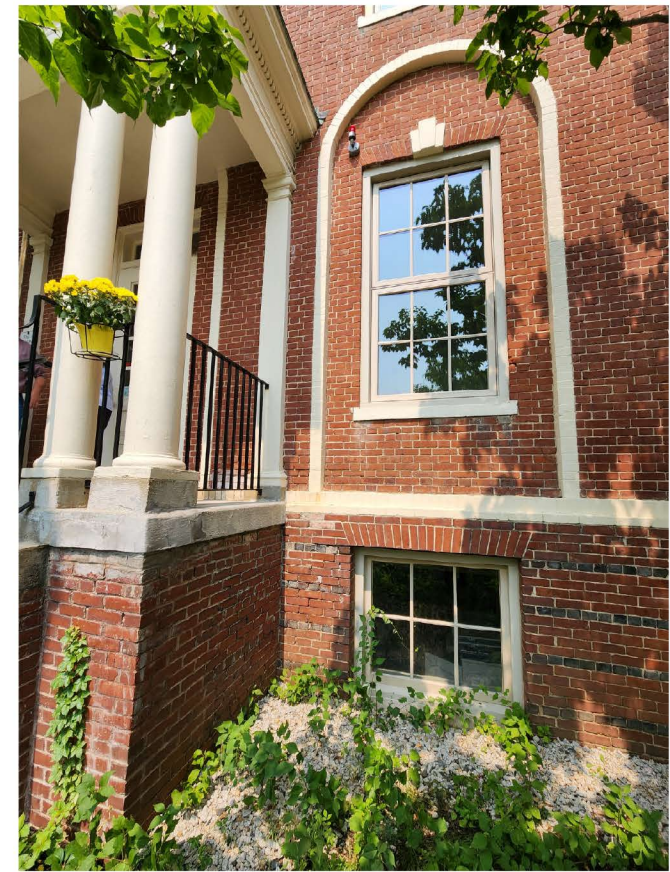
SOUTH ENTRY SIDE ACCESS POINT
