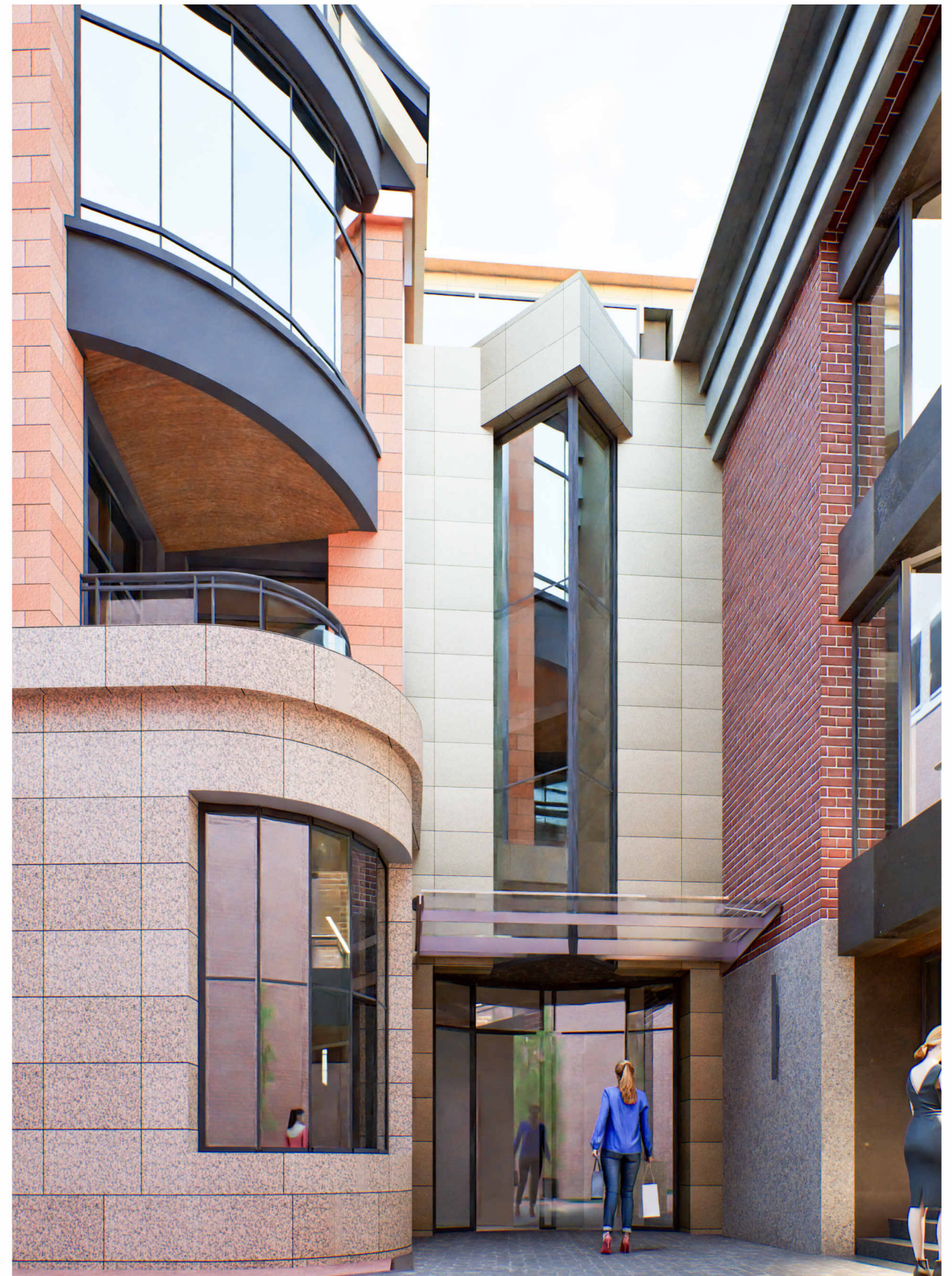
HAVEN COURT ENTRANCE
