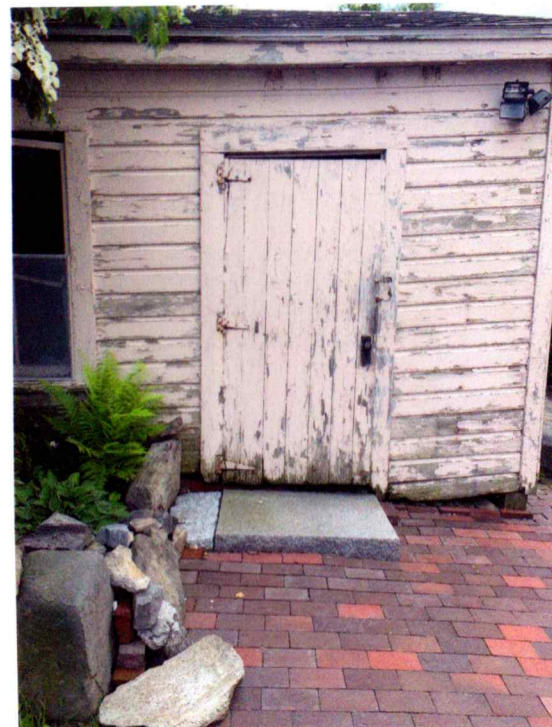
GARAGE EXIST LEFT SIDE
