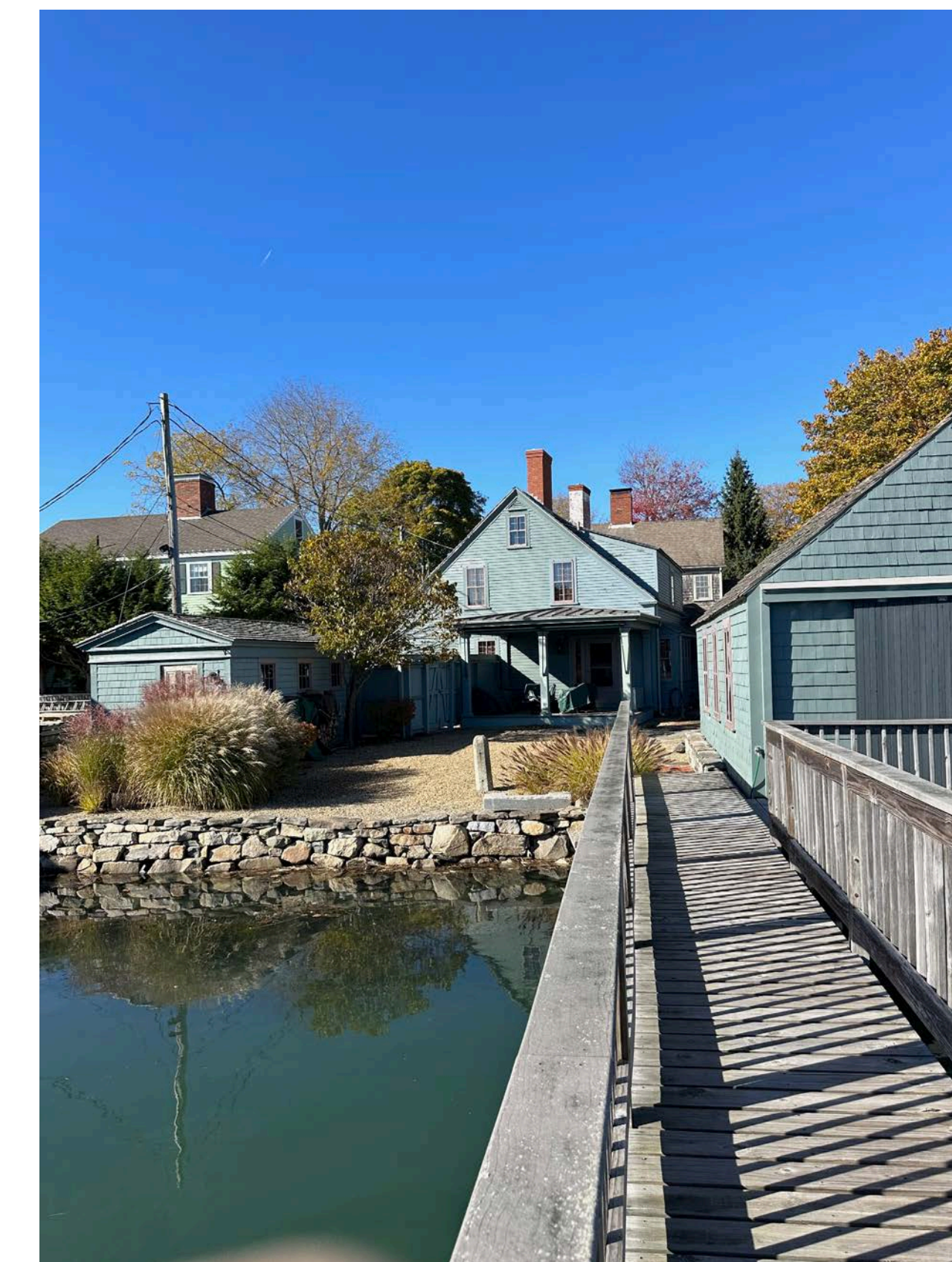
RIGHT VIEW FROM DOCK (EAST)
