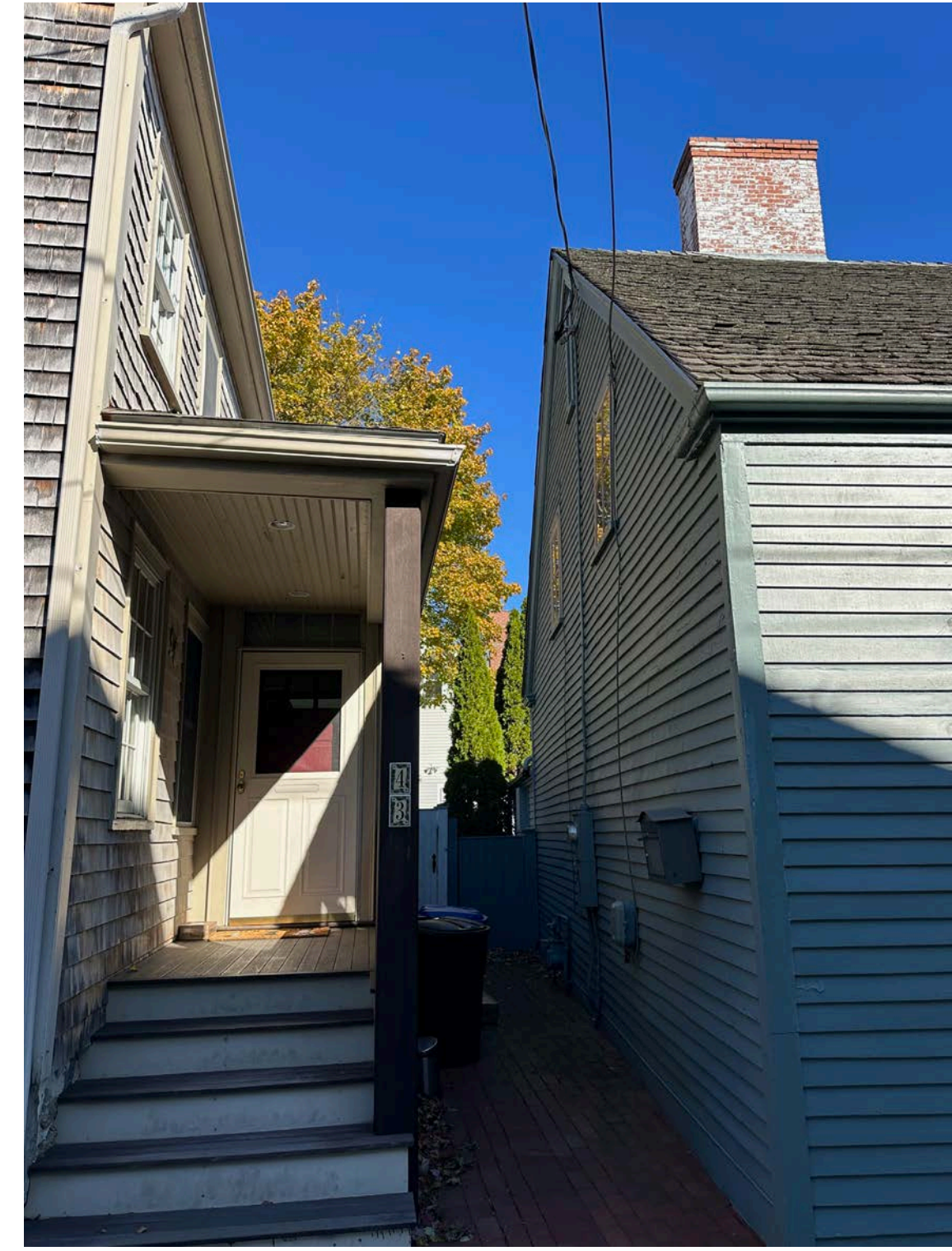
LEFT ALLEY (WEST)
