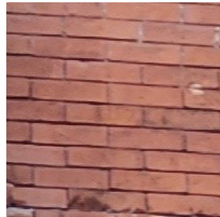
EXISTING BRICK - 15 CONGRESS STREET
