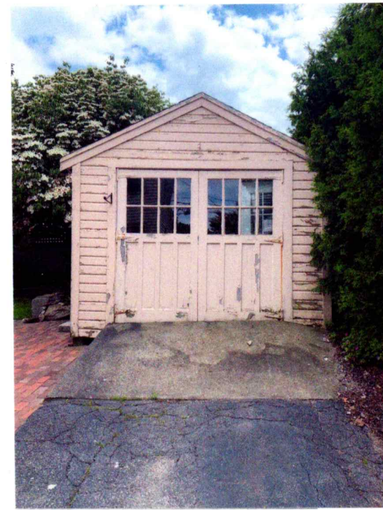
GARAGE EXIST FRONT
