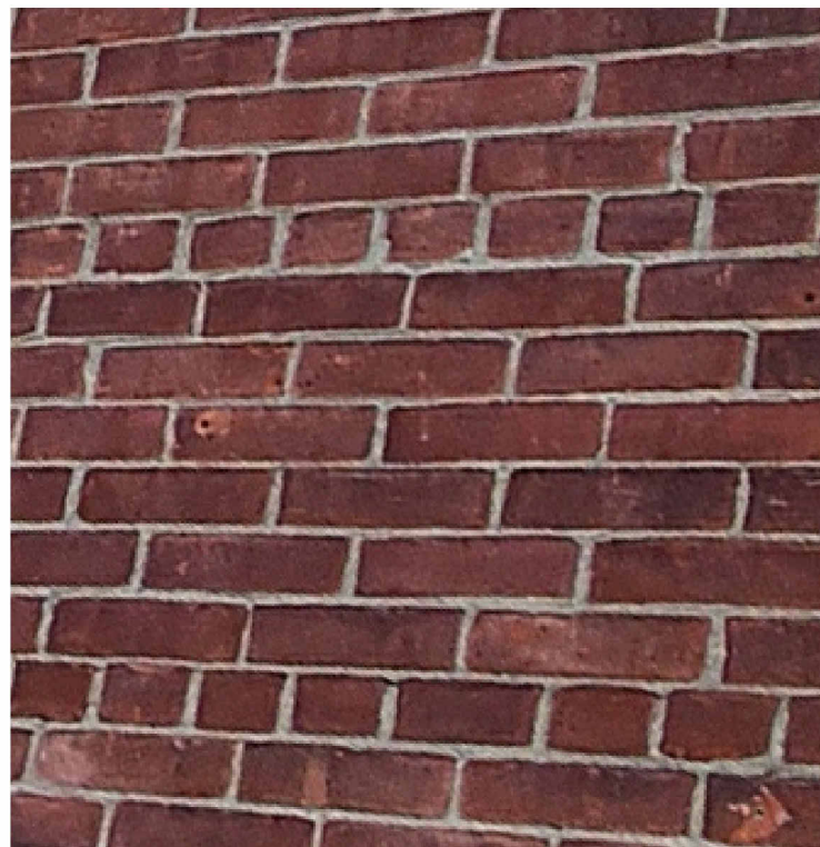
EXISTING BRICK - HAVEN COURT WEST
