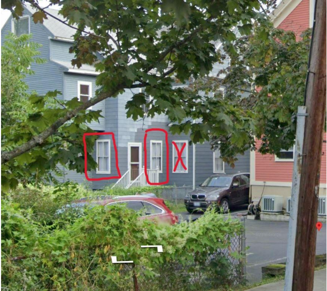
Windows to be replaced highlighted in red.
