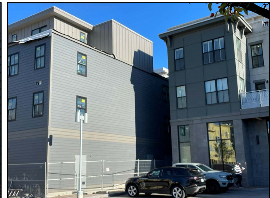
PERSPECTIVE OF SERVICE DECK FROM BRIDGE STREET (SCREENING HAS NOT BEEN INSTALLED YET)
