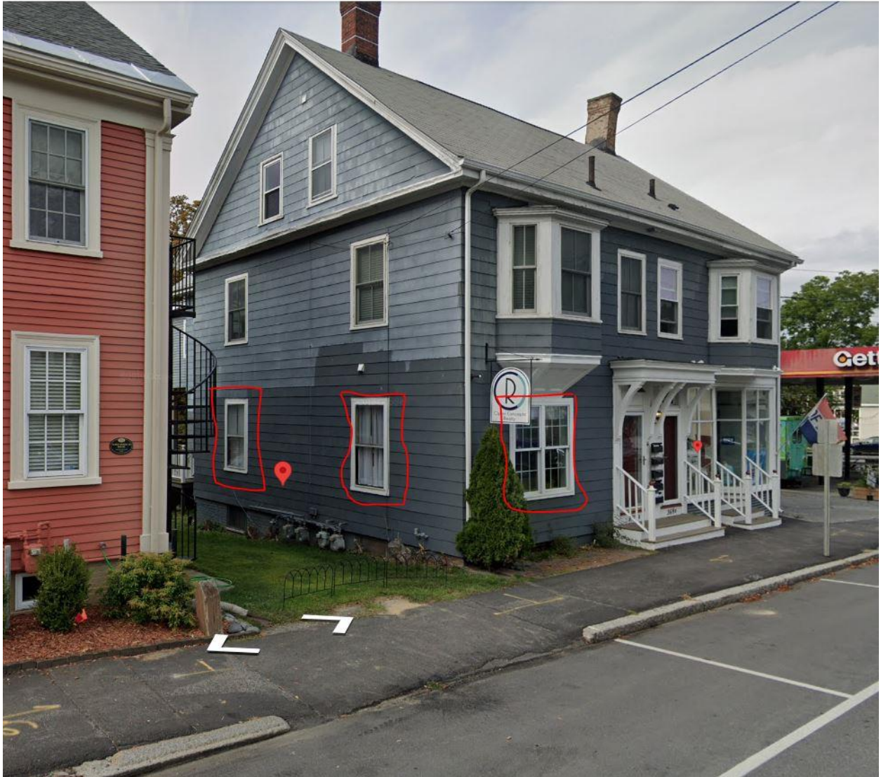
Windows to be replaced highlighted in red.
