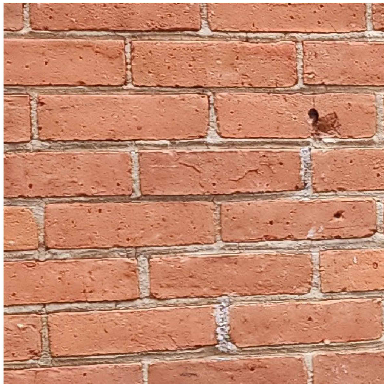
EXISTING BRICK - HAVEN COURT EAST
