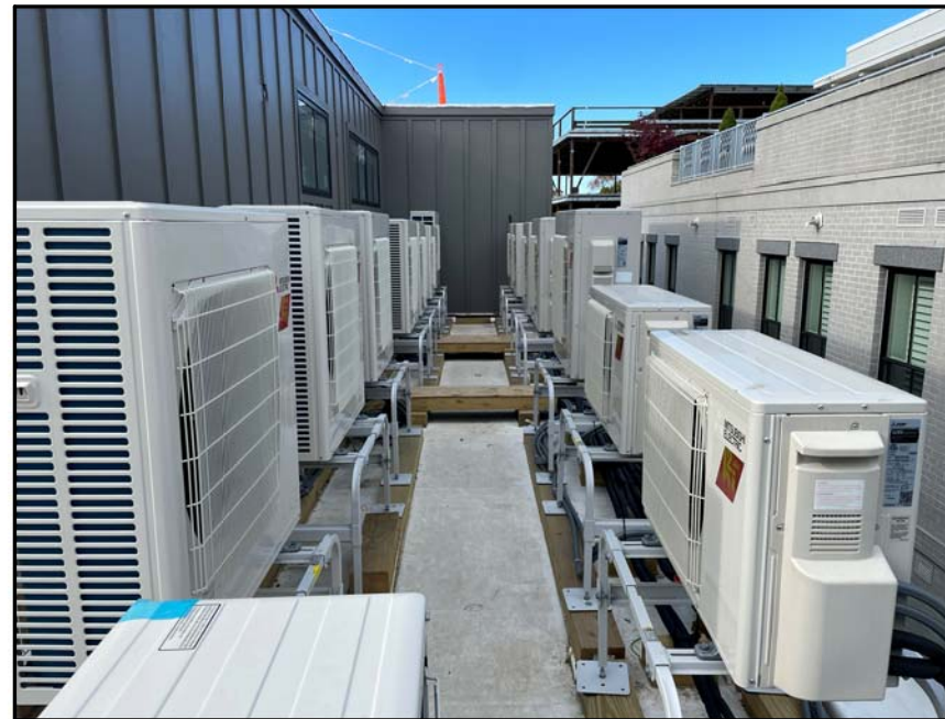
CONDENSERS ON SNOW STANDS, VIEW FROM SERVICE DECK
