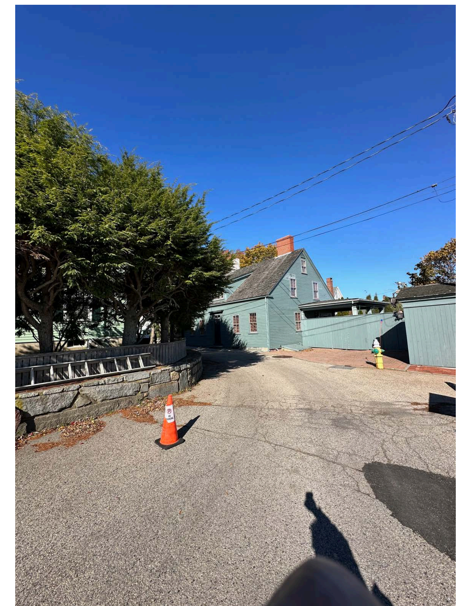
5 FROM PARKING LOT
