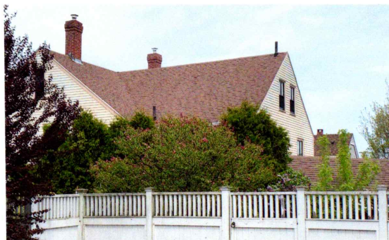
REAR ELEVATION FROM MARCY STREET
