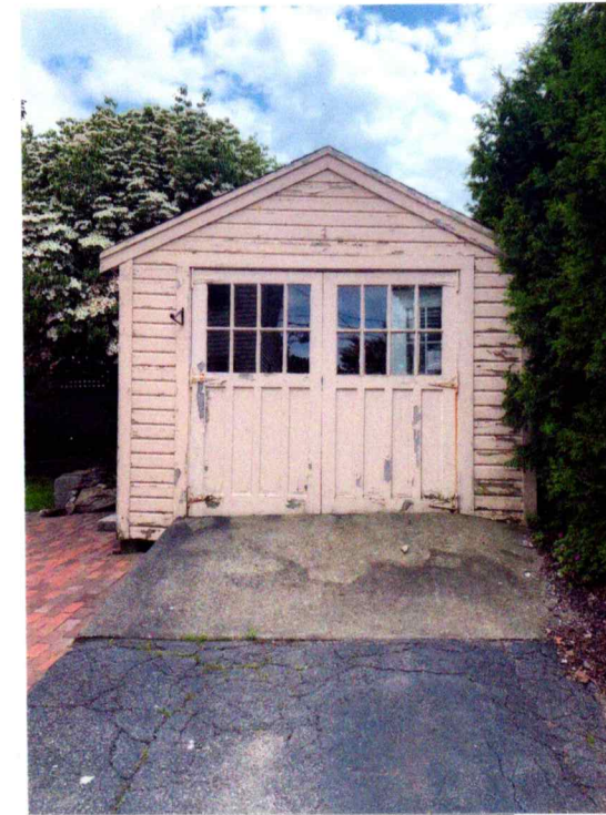
GARAGE EXIST FRONT
