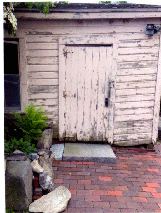
GARAGE EXIST LEFT SIDE
