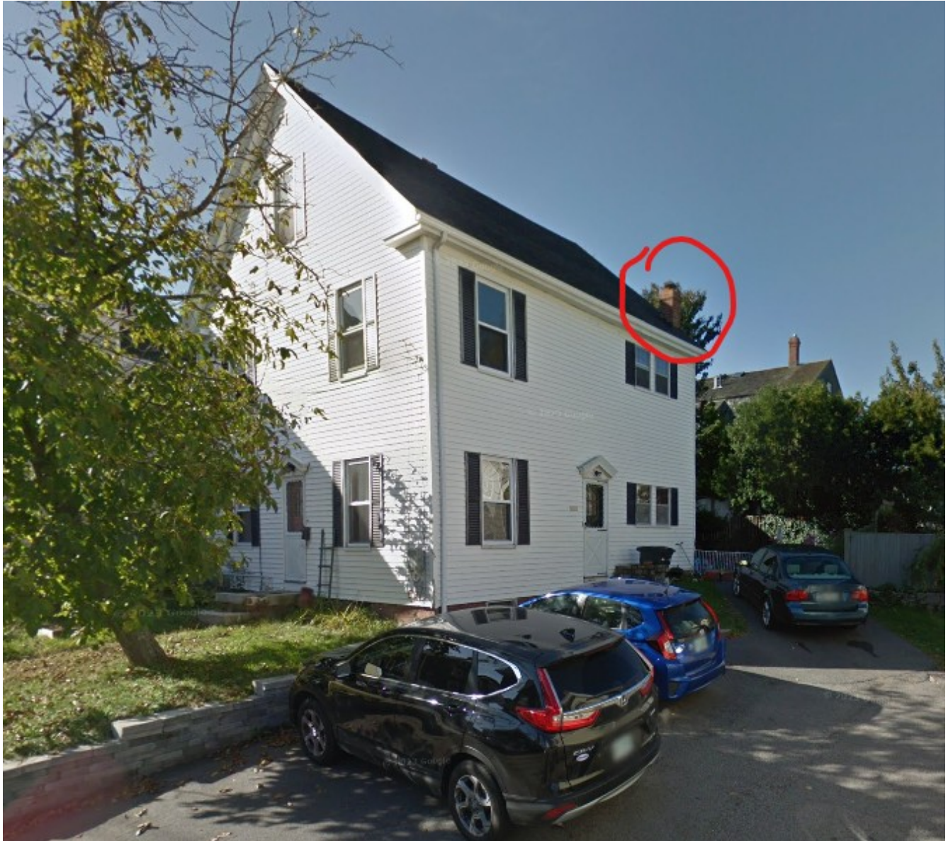
View of chimney from Marcy Street
