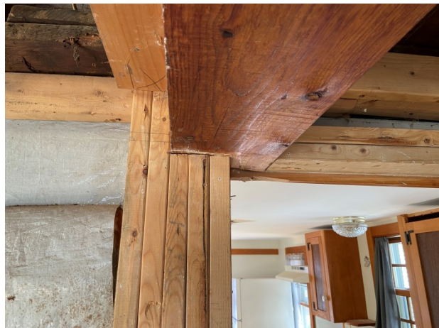
26-Timber beam end bearing
