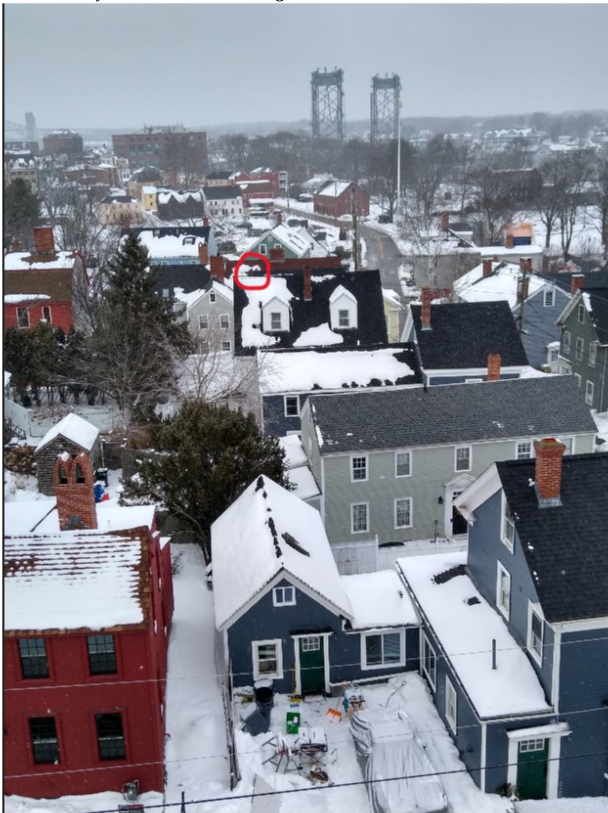
View of chimney from South Ward Meetinghouse
