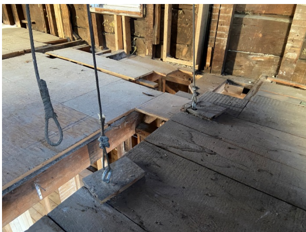
21-Cables supporting second floor
