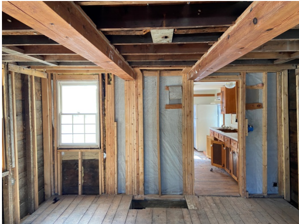
23-Second floor framing
