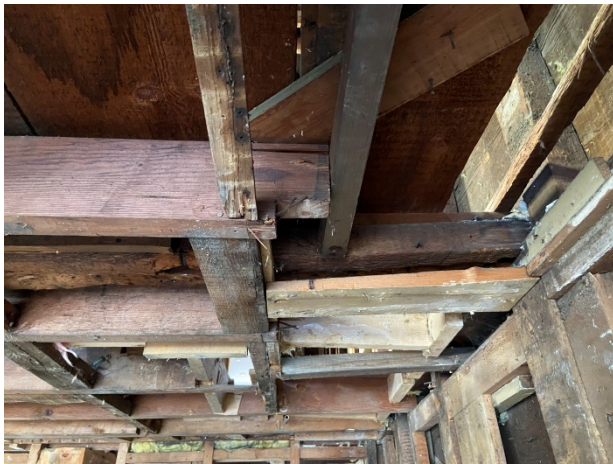
19-Front bay second floor framing
