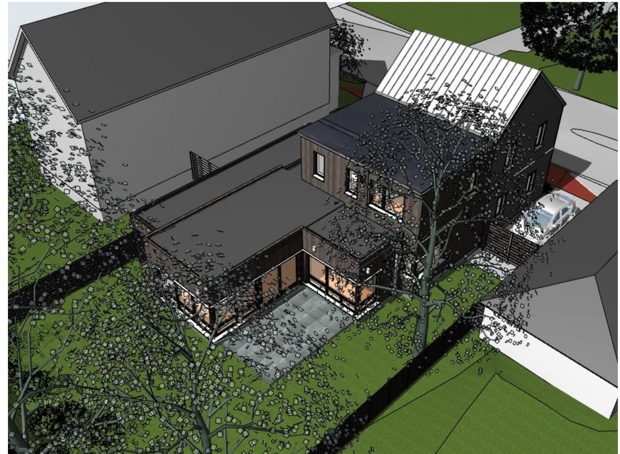
EXISTING CONDITIONS - AERIAL VIEW FROM SOUTH
