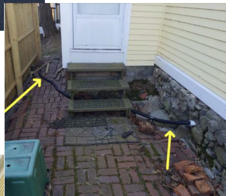
CLOSE UP OF EXISTING STAIR
