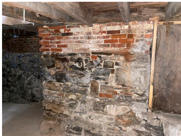
10-Basement looking east
