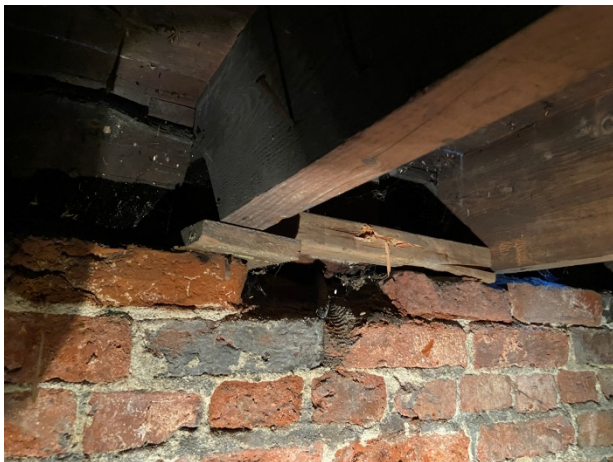
17-Detail of joist end bearing on shims
