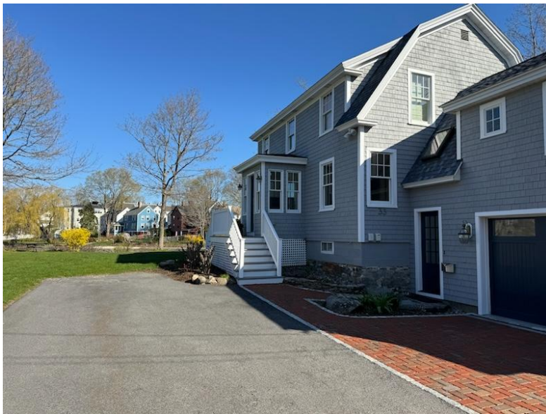
On Johnson Court in front of 33 Johnson. Main roof remains invisible. Garage roof is at a highly oblique angle.
