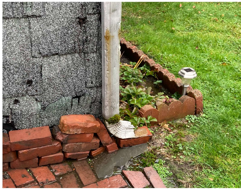
5) VIEW OF EXISTING FOUNDATION AT ATTACHED SHED
