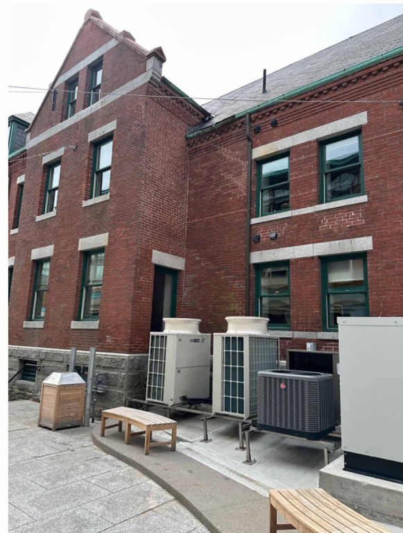
EXISTING COMPRESSOR TO BE COVERED
