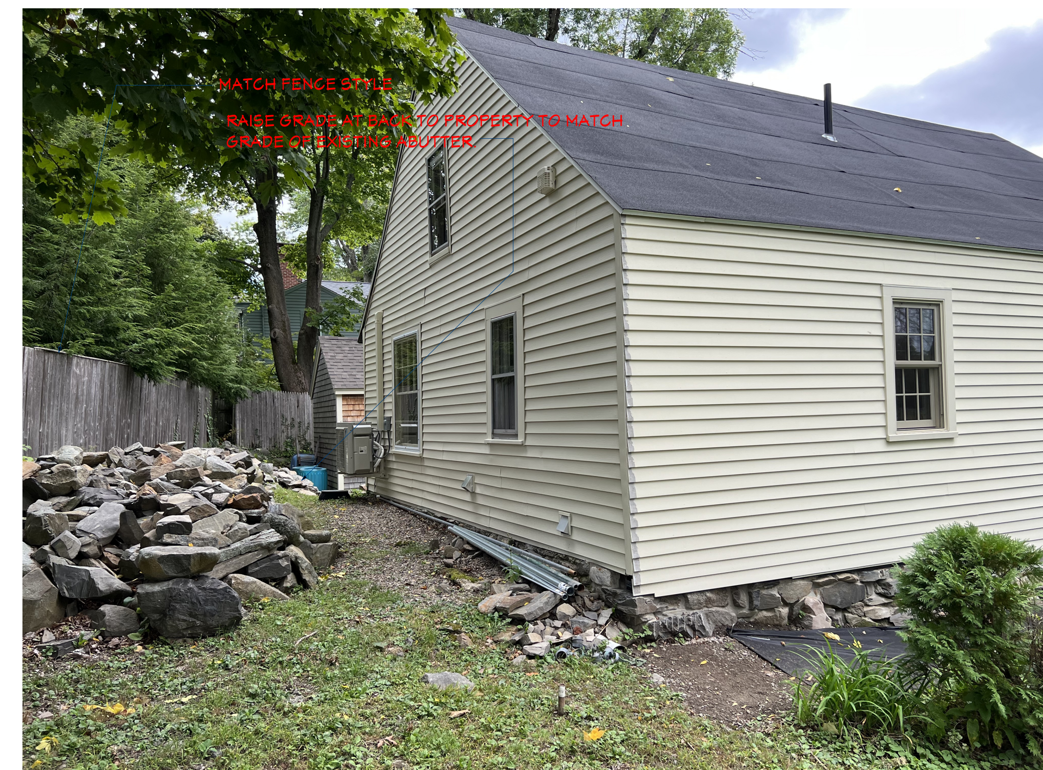
EXISTING BACK GRADE & FENCE
