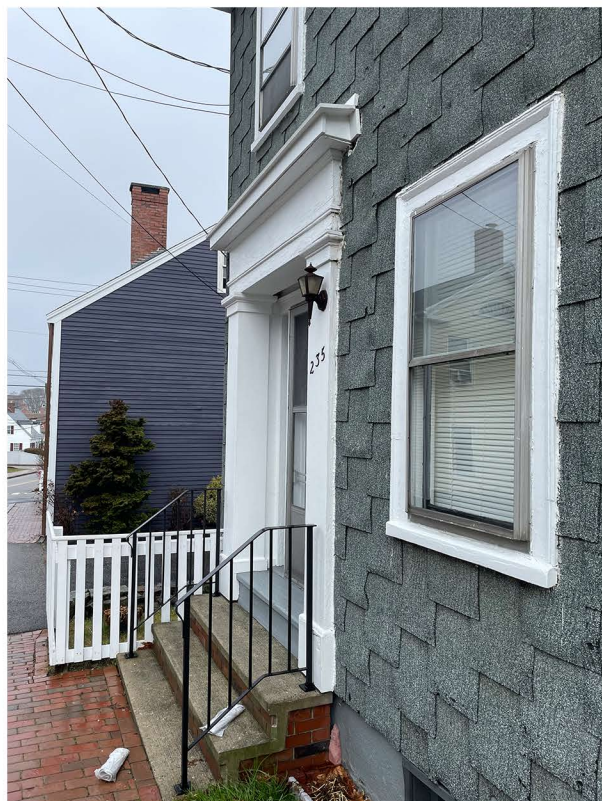
4) VIEW OF EXISTING WINDOW CASING
