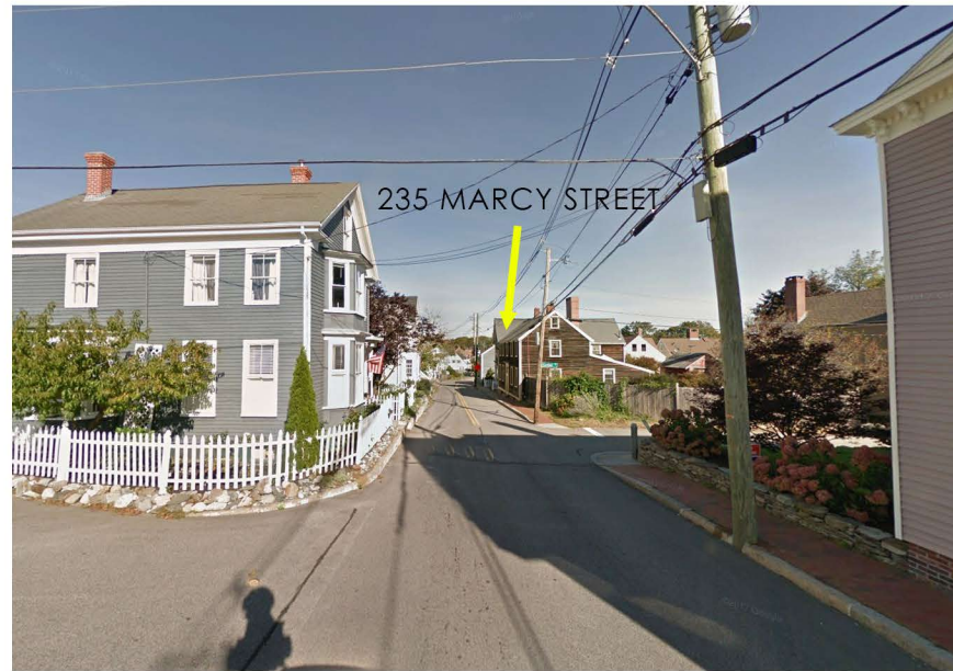
3) VIEW FROM SOUTH OF MARCY STREET
