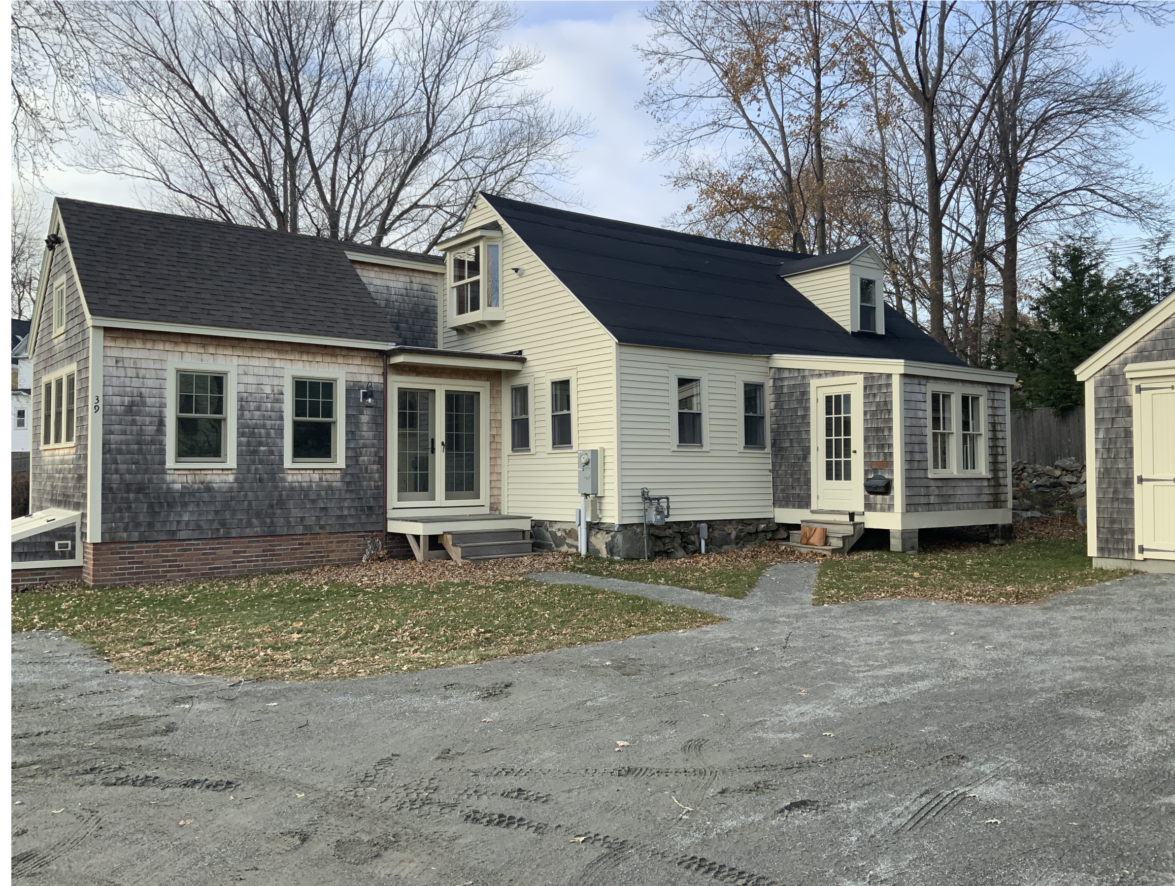
EXISTING FRONT HOUSE
