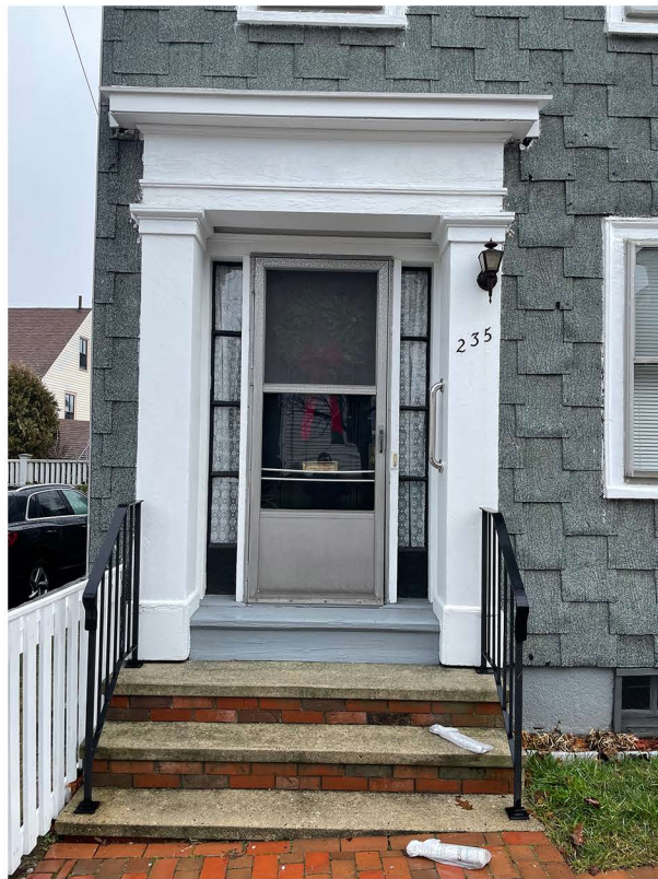
1) VIEW OF EXISTING FRONT ENTRY
