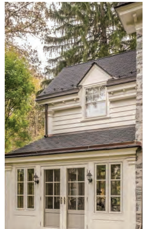
Raised panel with shed above
