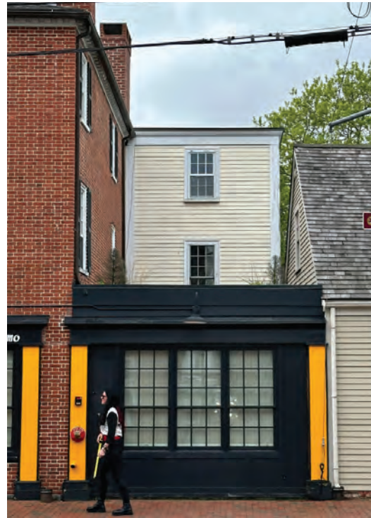
Existing Roof - For slanted across
