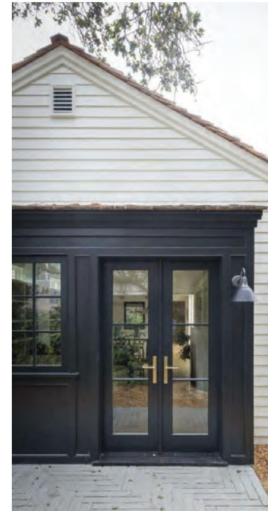
Raised panel with door wood clad above
