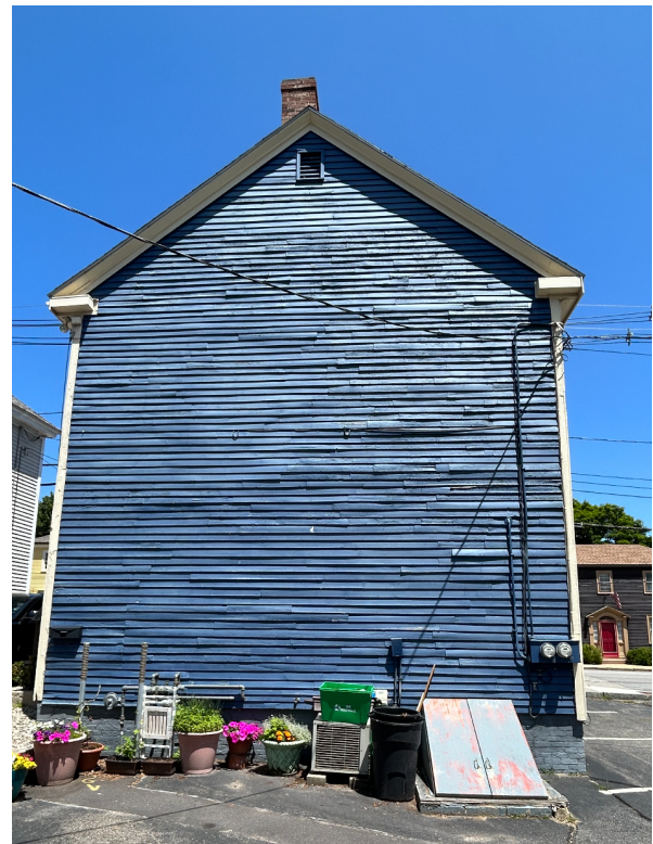
Rear facade abutting neighbor on Dennett St
