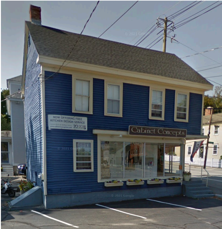
Facade facing Dennett Street
