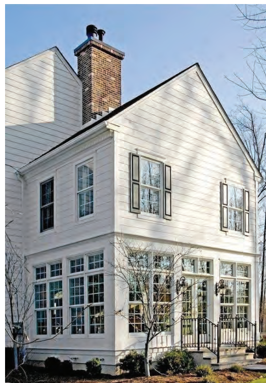
Raised panel wood clad panel above
