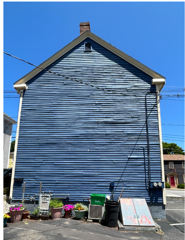
Rear facade abutting neighbor on Dennett St
