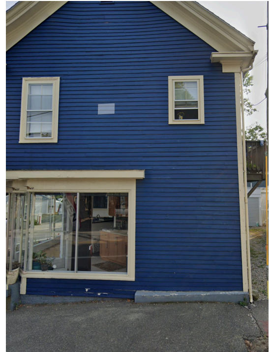
Facade facing Maplewood Ave
