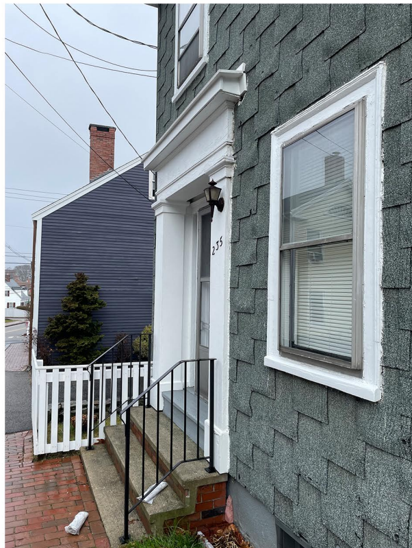
4) VIEW OF EXISTING WINDOW CASING
