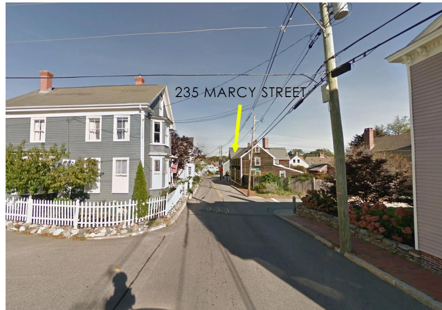
3) VIEW FROM SOUTH OF MARCY STREET
