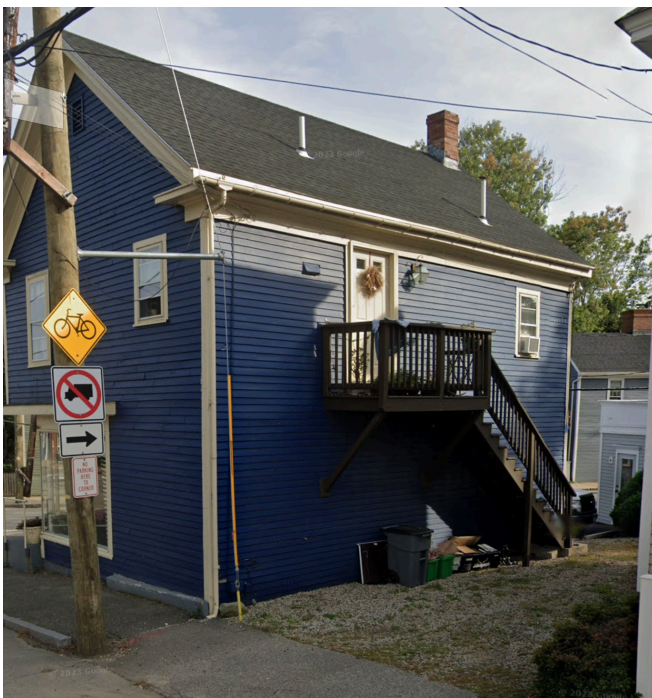
Facade view from Maplewood
