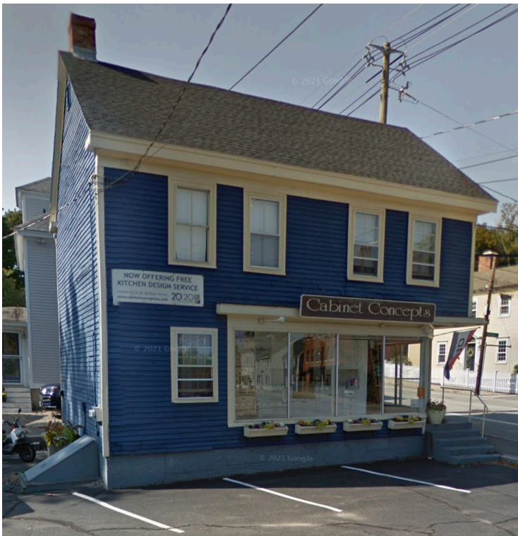
Facade facing Dennett Street
