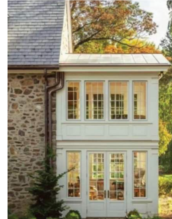
Raised panel facade abutting masonry
