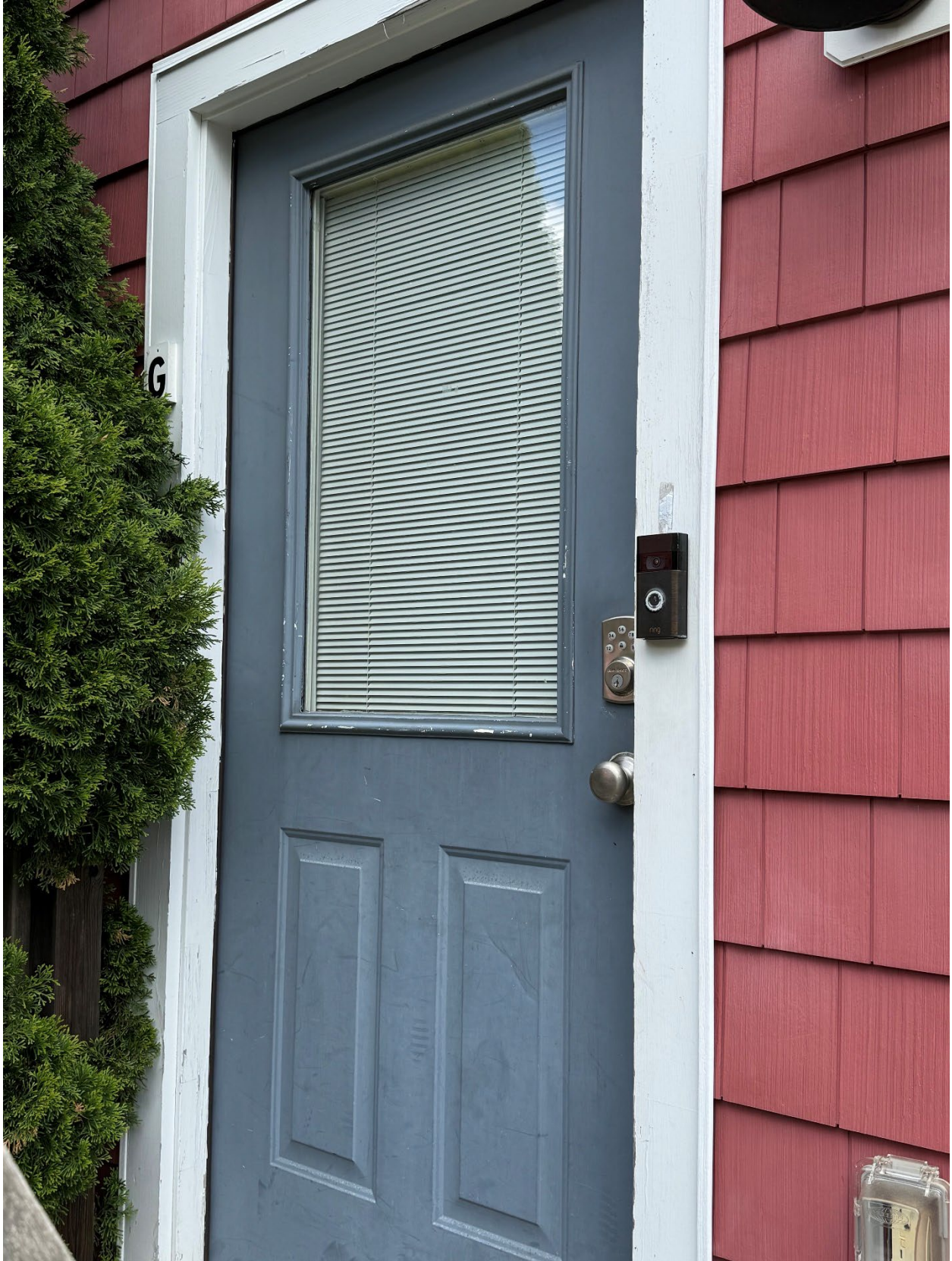
Existing door(s) on the rest of the structure.
