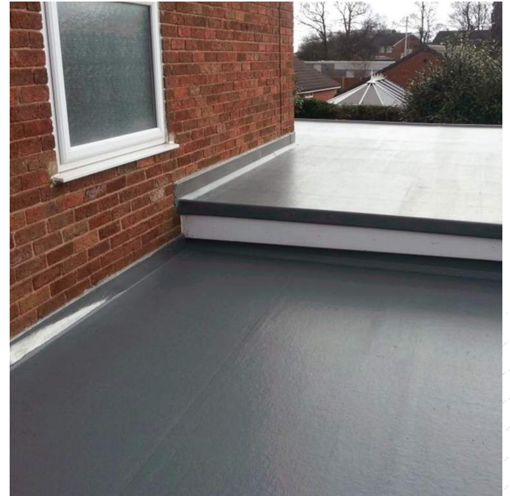
EPDM Rubber membrane roof
