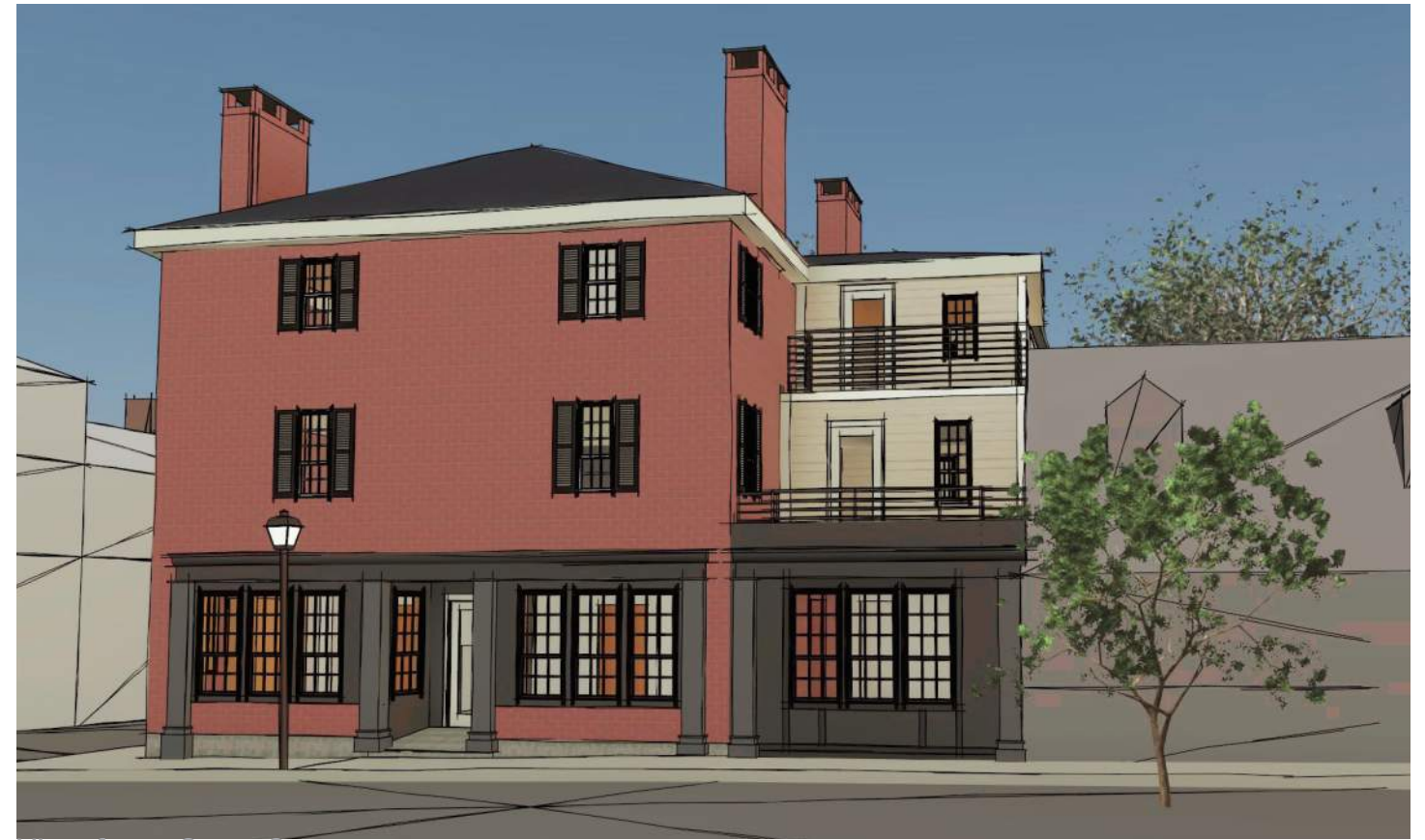
View from State Street
