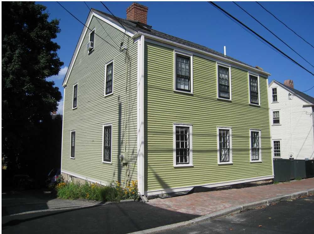
Front and Left Side View – Original House
