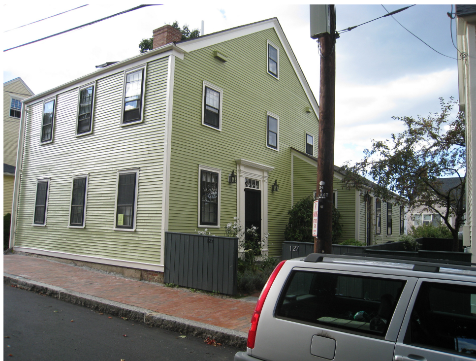
Front and Right Side View – Original House w/ peek at addition
