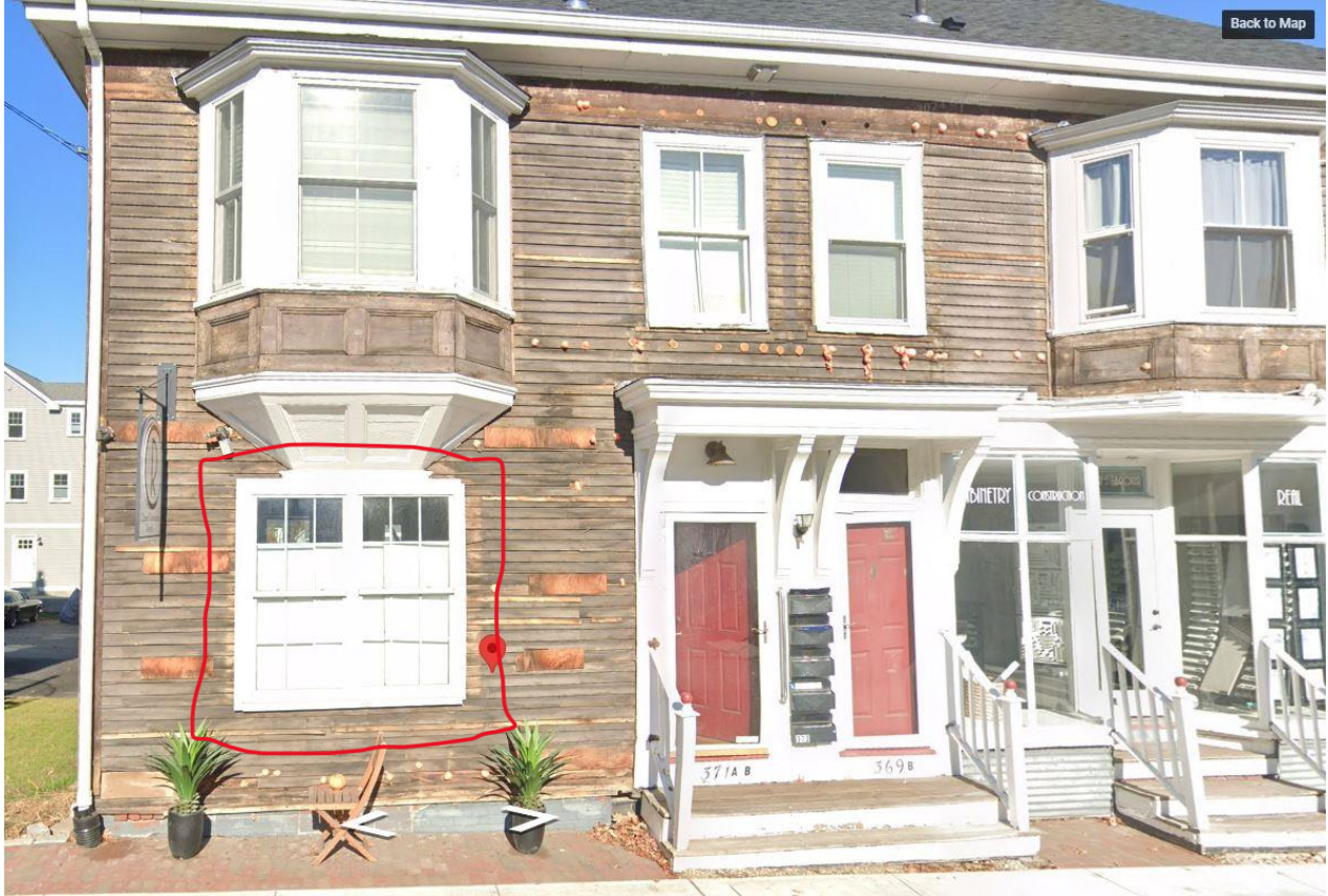
Current conditions, double window highlighted is to be replaced.
