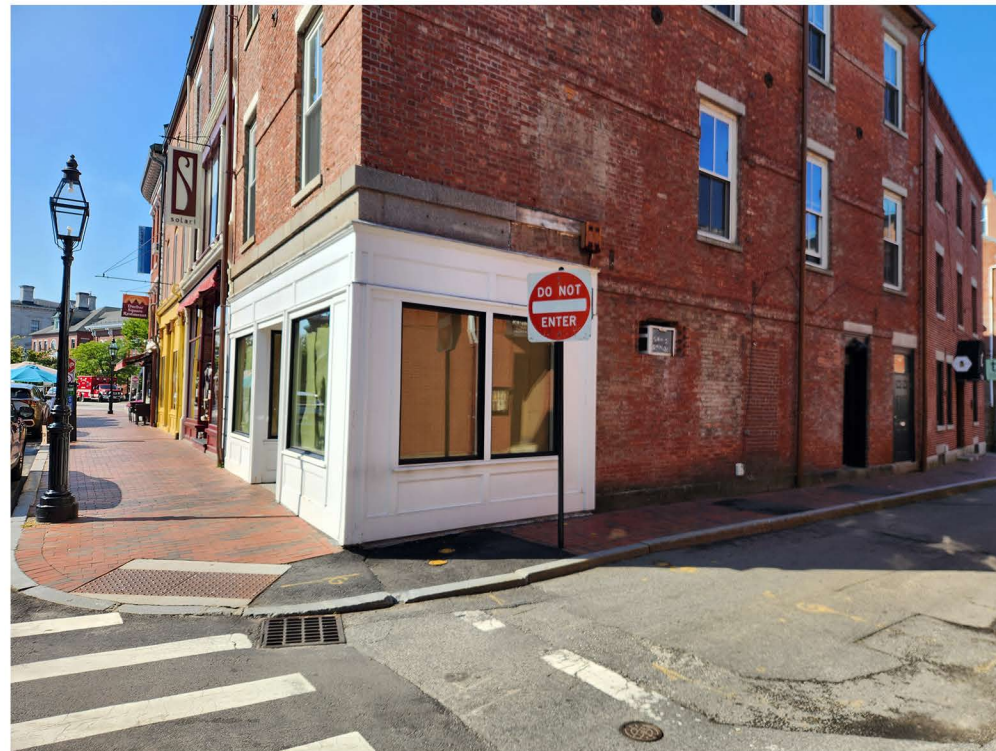
VIEW FROM MARKET STREET AND LADD STREET INTERSECTION
