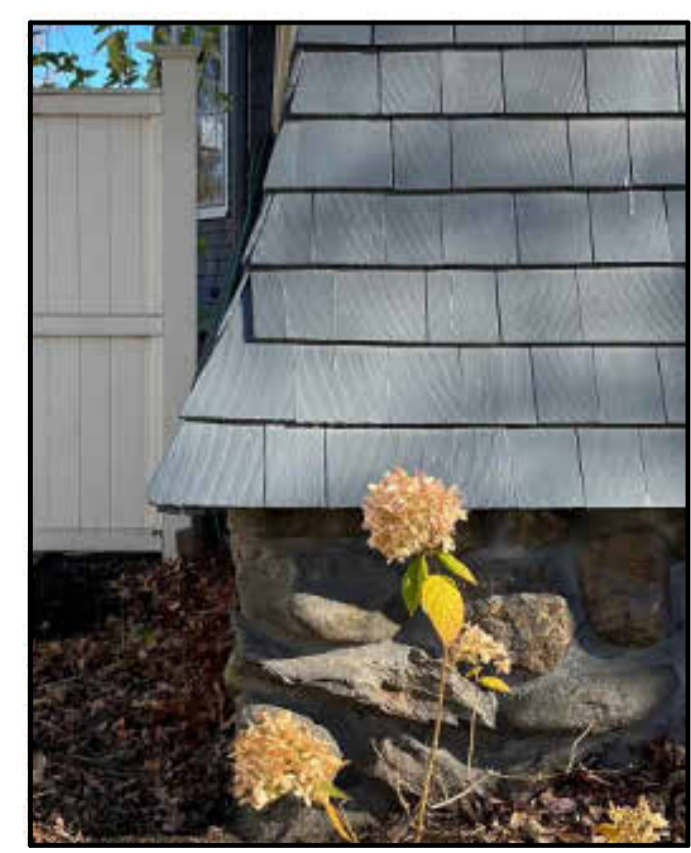
MAIN HOME - BASE WALL SWEEP
