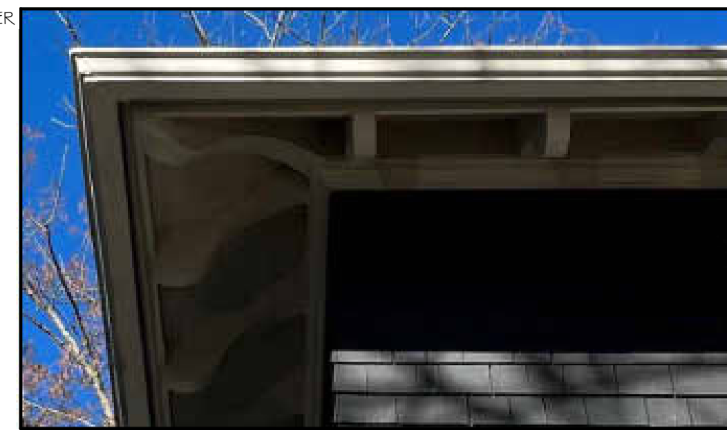
MAIN HOME - RAFTER TAILS
