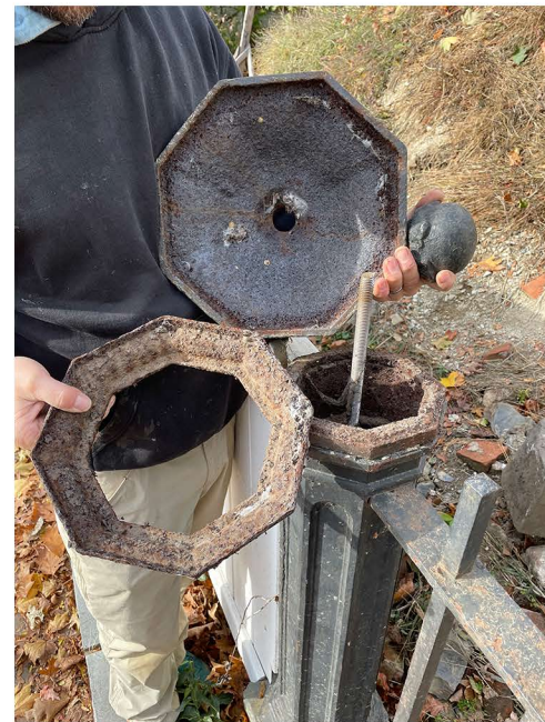
VIEW OF EXISTING IRON POSTS
