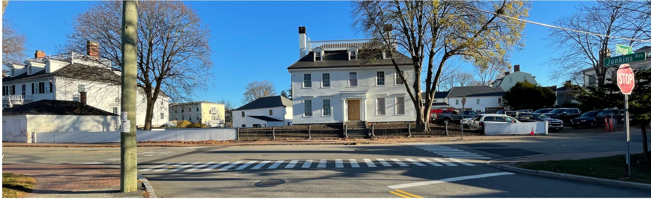
VIEW OF EXISTING FRONT FENCES & GATE
