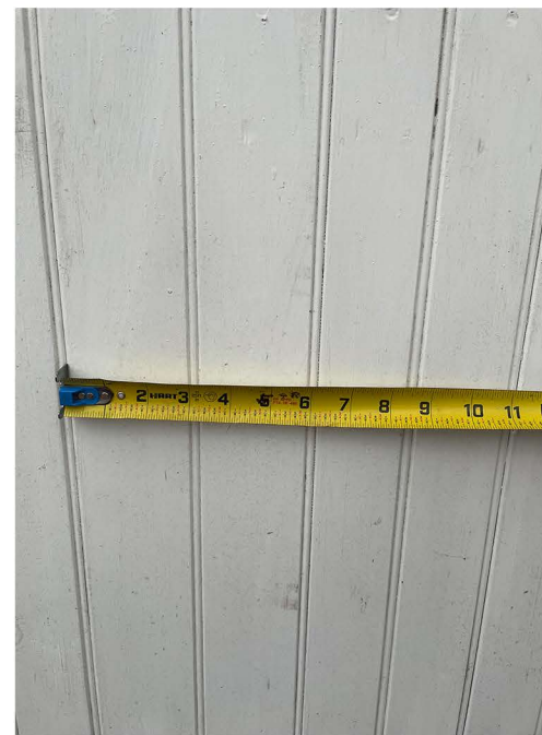
EXISTING LANGDON FENCE
