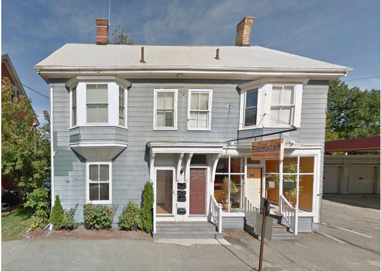
Façade prior to double window being installed.
