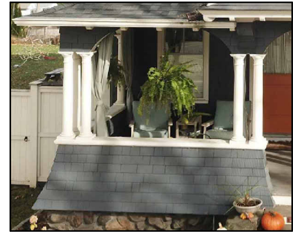
MAIN HOME - HALF WALL @ DECK
