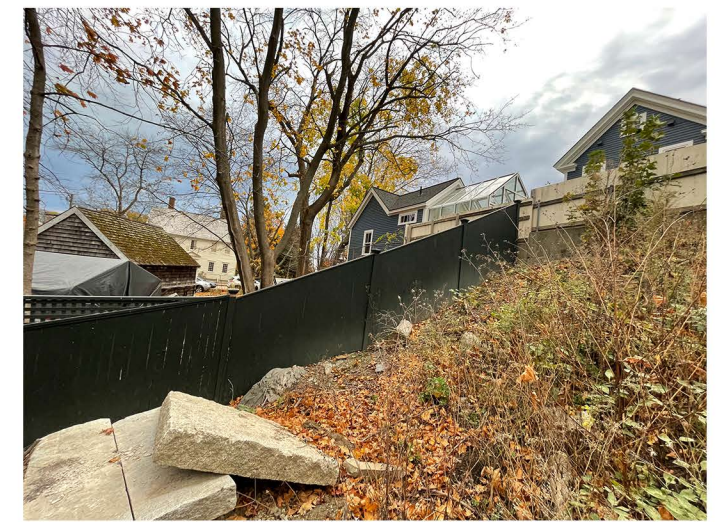
VIEW OF EXISTING FENCE
