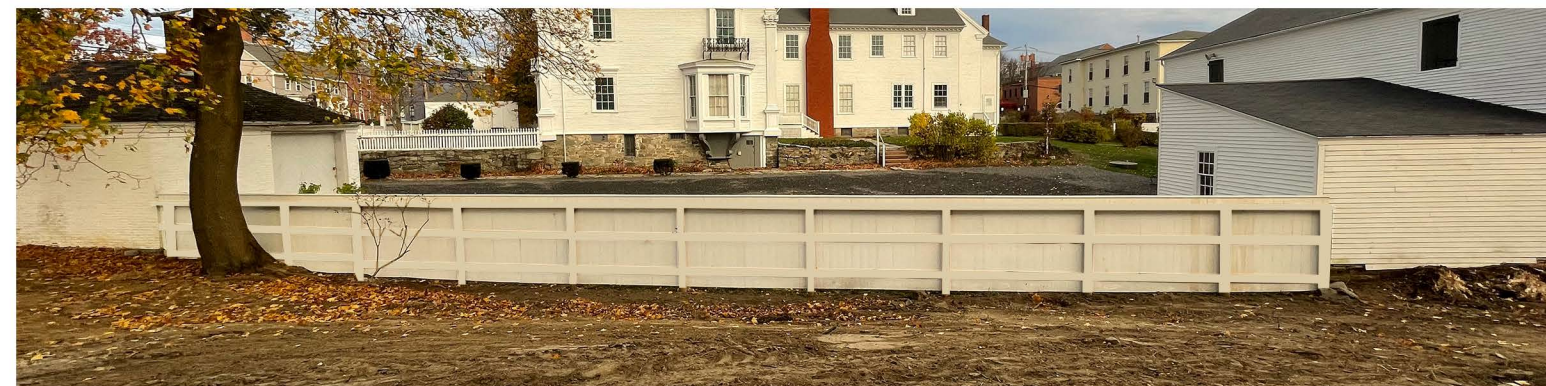
VIEW OF EXISTING FENCE TO REMAIN
