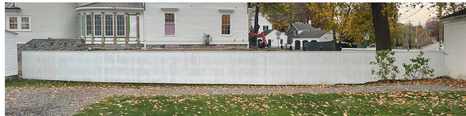
VIEW OF EXISTING FENCE TO REMAIN
