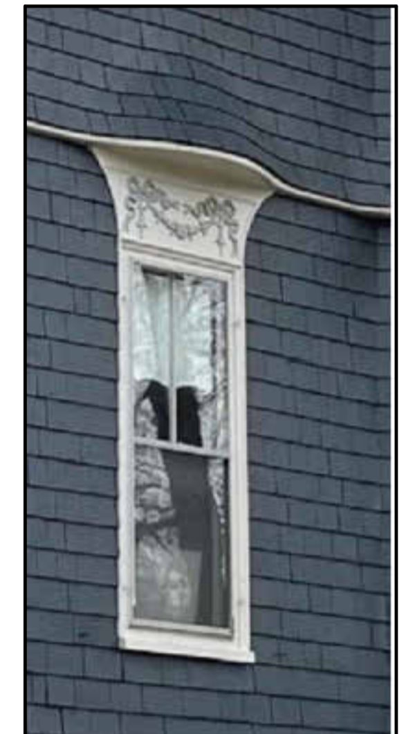
MAIN HOME - MID-WALL / WINDOW SWEEP
