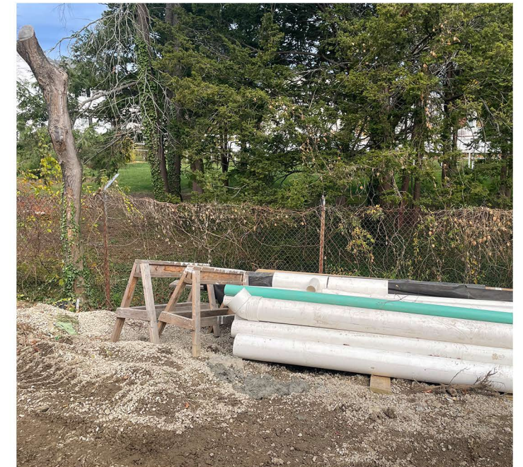
VIEW OF EXISTING CHAINLINK FENCE
