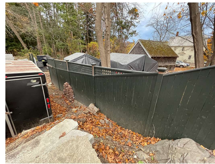
VIEW OF EXISTING FENCE
