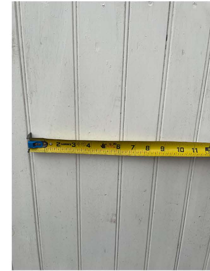
EXISTING LANGDON FENCE
