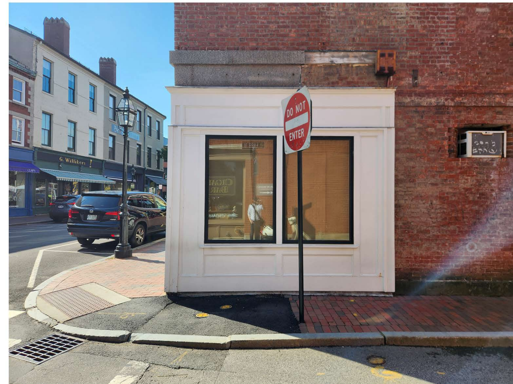
VIEW FROM LADD STREET
