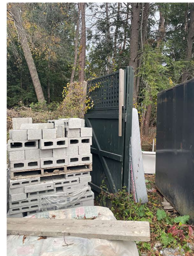
VIEW OF EXISTING GATE
