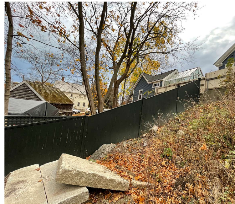
VIEW OF EXISTING WOOD FENCE
