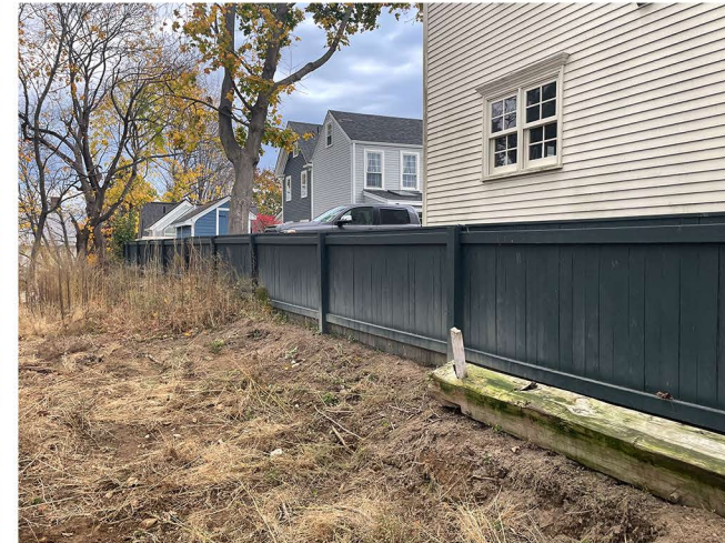
VIEW OF EXISTING WOOD FENCE
