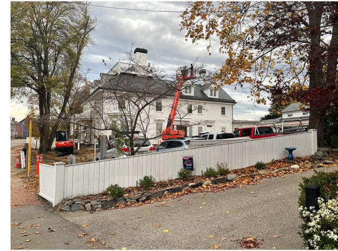
VIEW OF EXISTING WOOD FENCE
