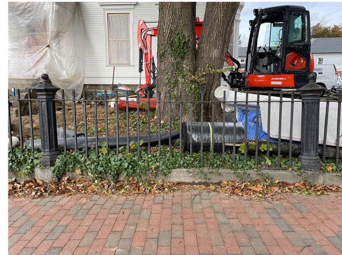
EXISTING IRON FENCE
