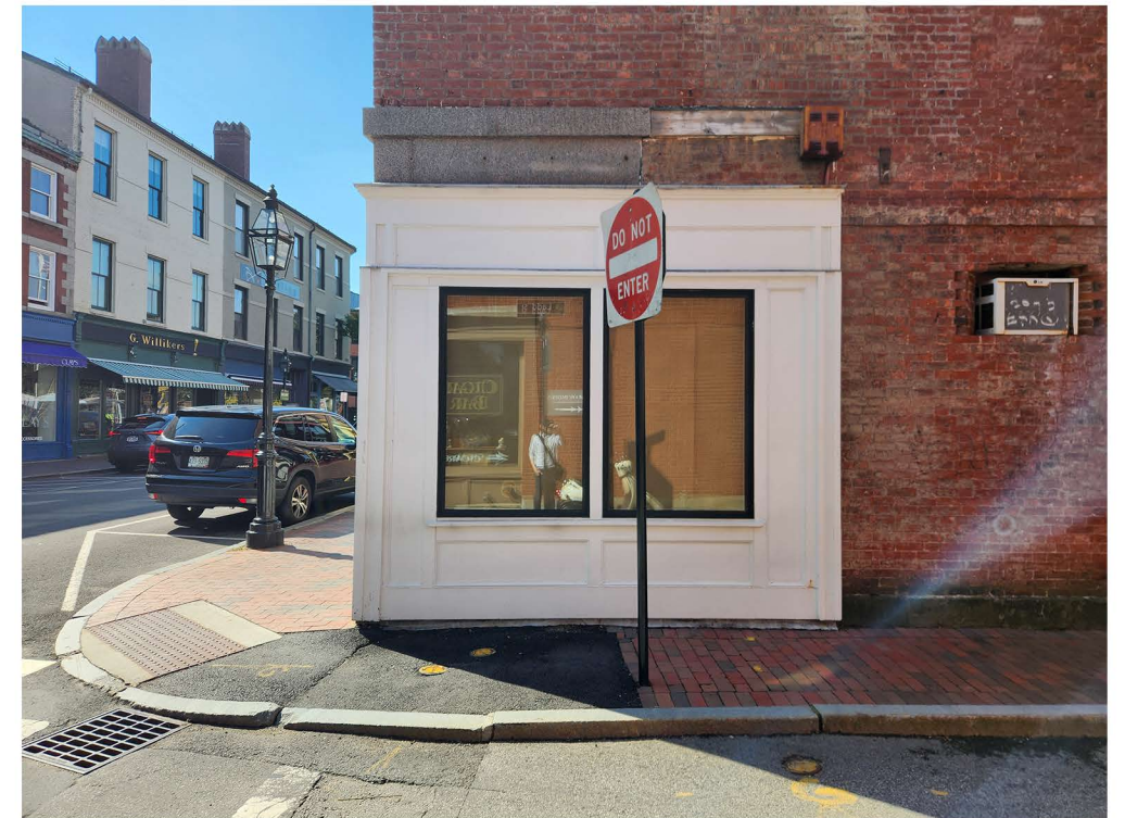
VIEW FROM LADD STREET
