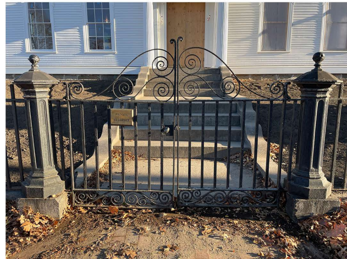
EXISTING FRONT GATE
