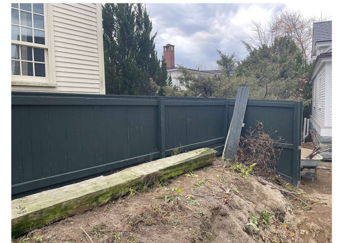
VIEW OF EXISTING WOOD FENCE
