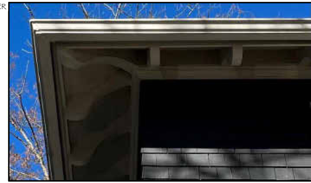
MAIN HOME - RAFTER TAILS
