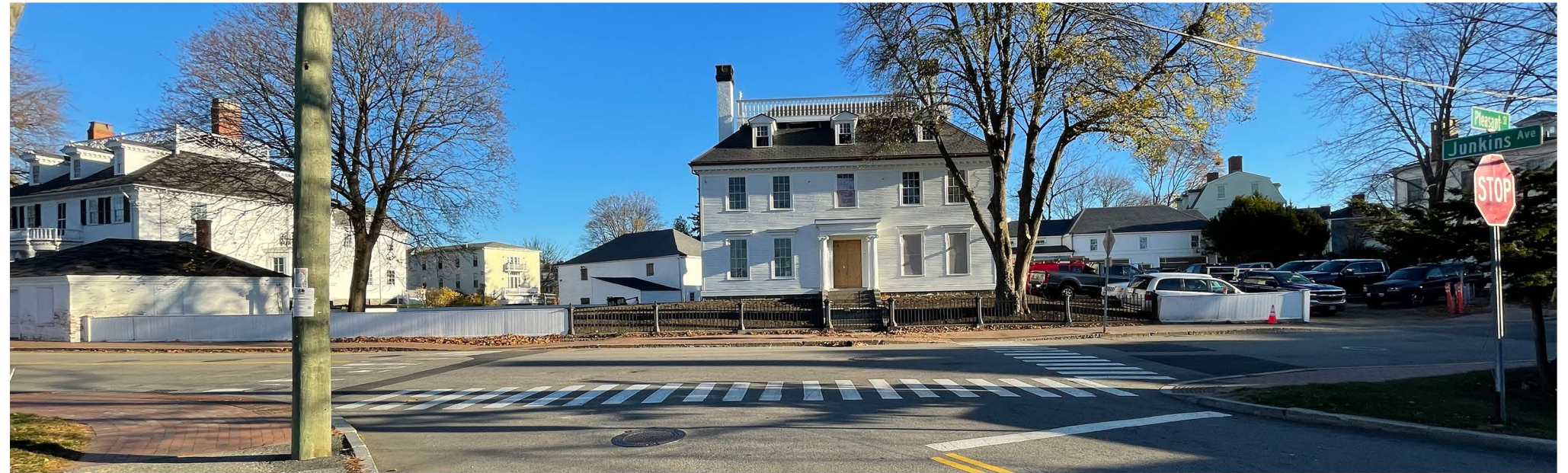
VIEW OF EXISTING FRONT FENCES & GATE
