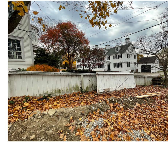
VIEW OF EXISTING WOOD FENCE
