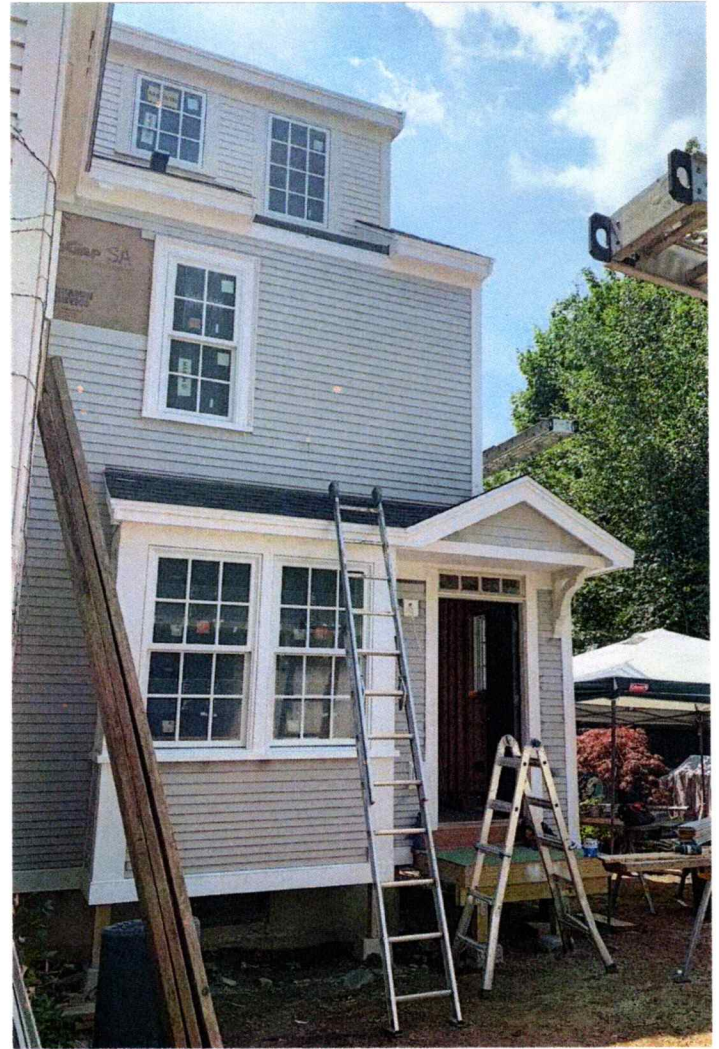
VIEW OF REAR SIDE ENTRY
