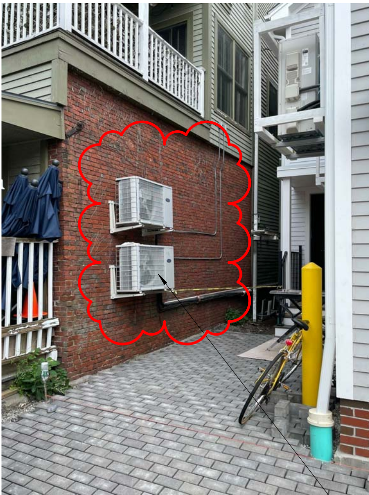
EXISTING WALL MOUNTED CONDENSER UNITS AND REFRIGERANT LINES TO BE REMOVED
