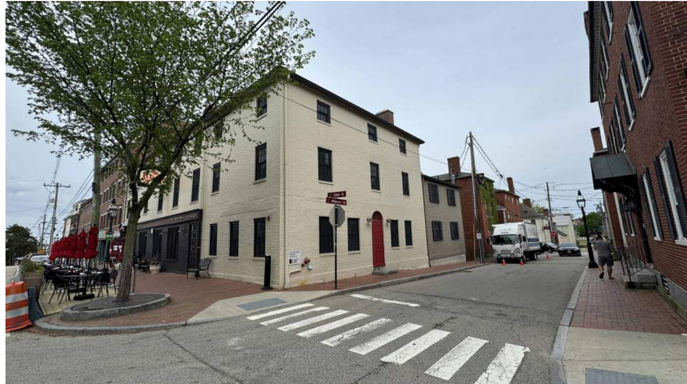
VIEW DOWN ATKINSON STREET
