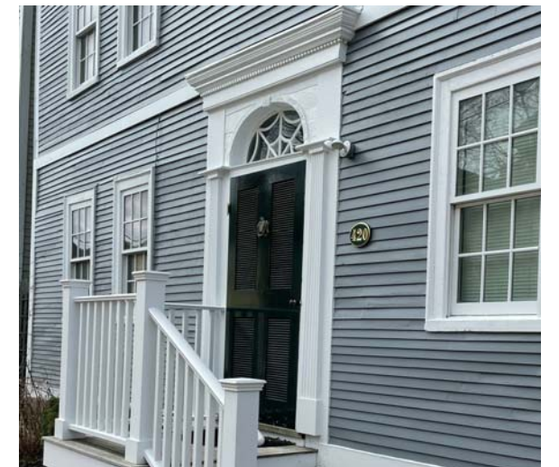
DESIGN INTENT: PROPOSED WOOD EXTERIOR ENTRY DOOR TO BE FOUR PANEL SIMILAR TO FRONT ENTRY DOOR WITH TWO LITES
