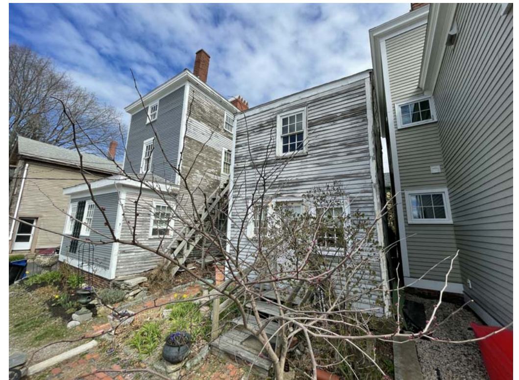
VIEW OF EXISTING SOUTHEAST ADDITION
