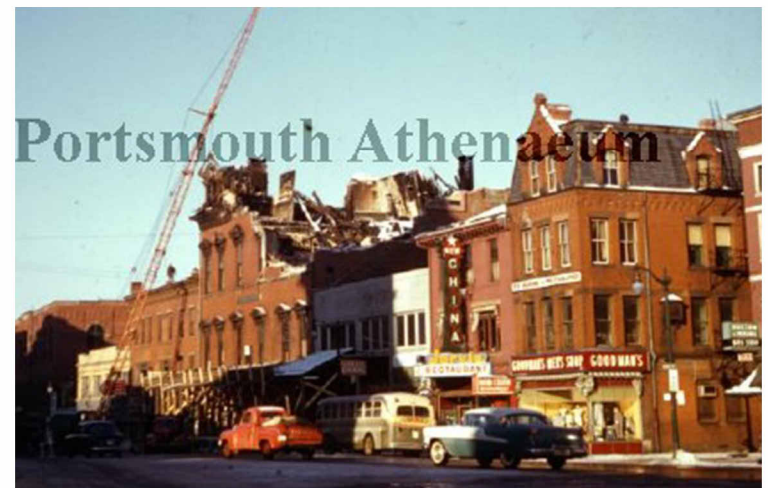
DEMOLITION AFTER THE FIRE
