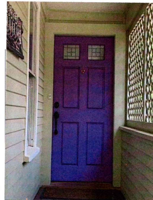
REAR ENTRY DOOR
