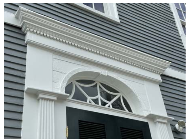
DESIGN INTENT: PROPOSED REAR HALF ROUND WINDOW TO BE SIMILAR TO FRONT DOOR TRANSOM
