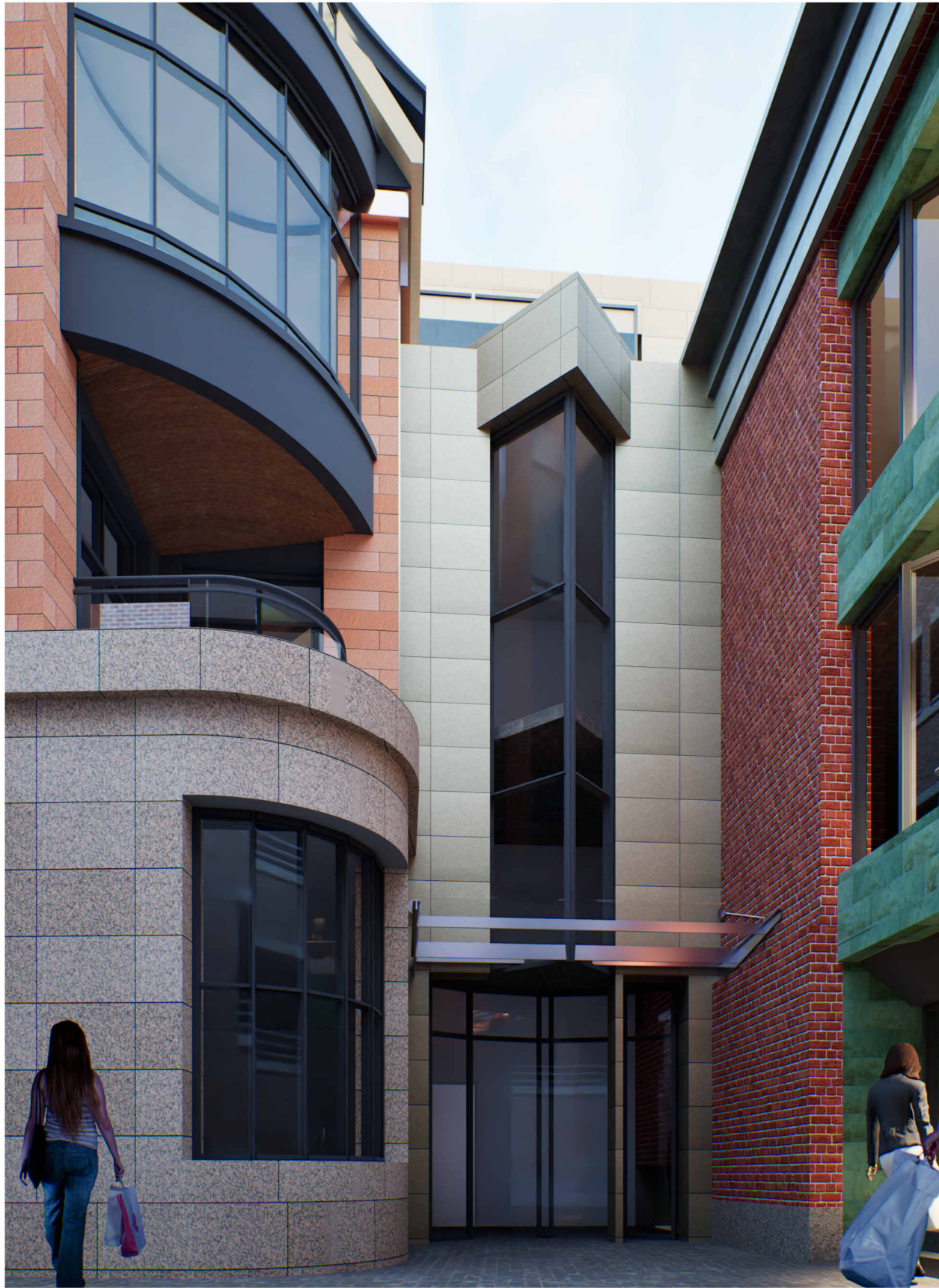
HAVEN COURT ENTRANCE
