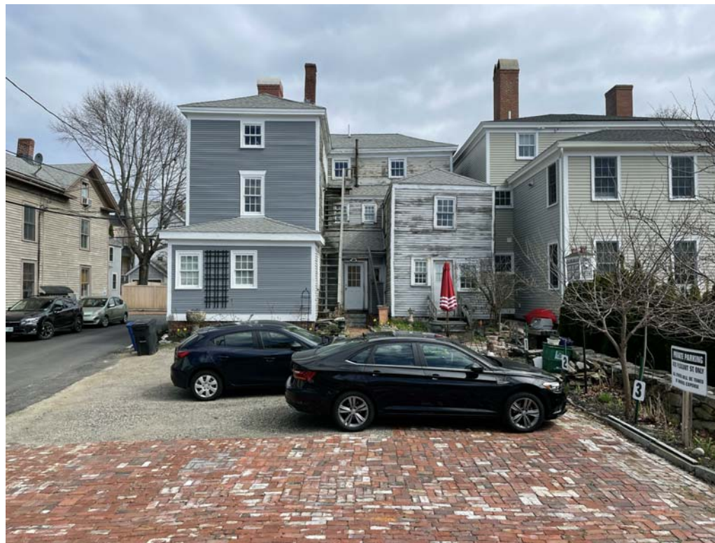
VIEW FROM 420 PLEASANT STREET PARKING LOT
