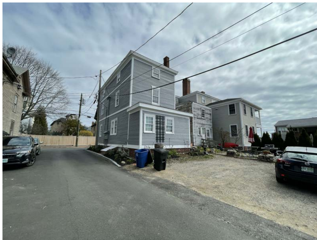
REAR OF BUILDING FROM FRANKLIN STREET
