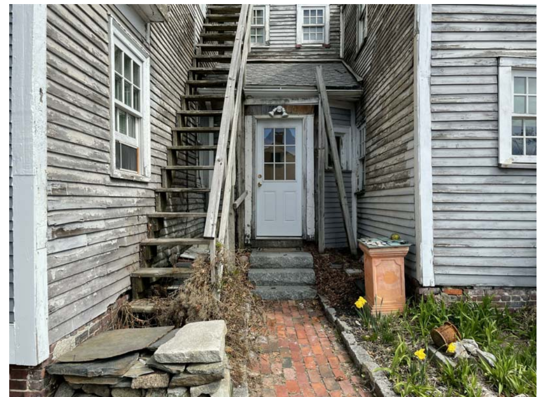
EXISTING REAR ENTRY
