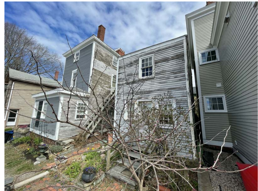
VIEW OF EXISTING SOUTHEAST ADDITION
