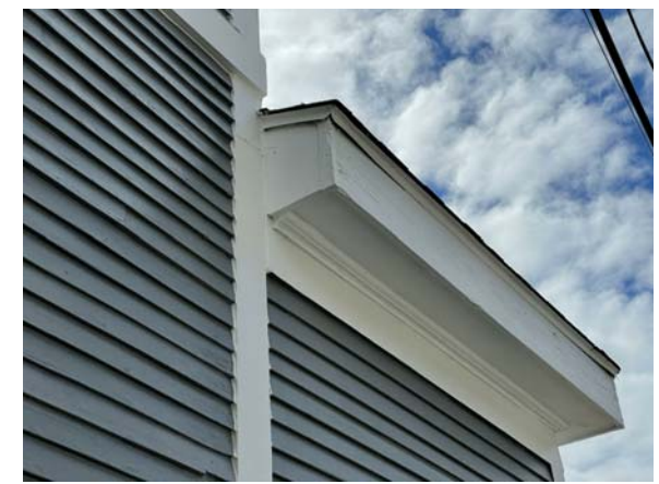
DESIGN INTENT: MATCH EXISTING HIP ROOF EAVE AND SOFFIT WOOD TRIM, WOOD CORNERBOARDS AND OTHER WOOD TRIM AT PROPOSED ADDITIONS
