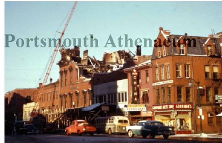
DEMOLITION AFTER THE FIRE
