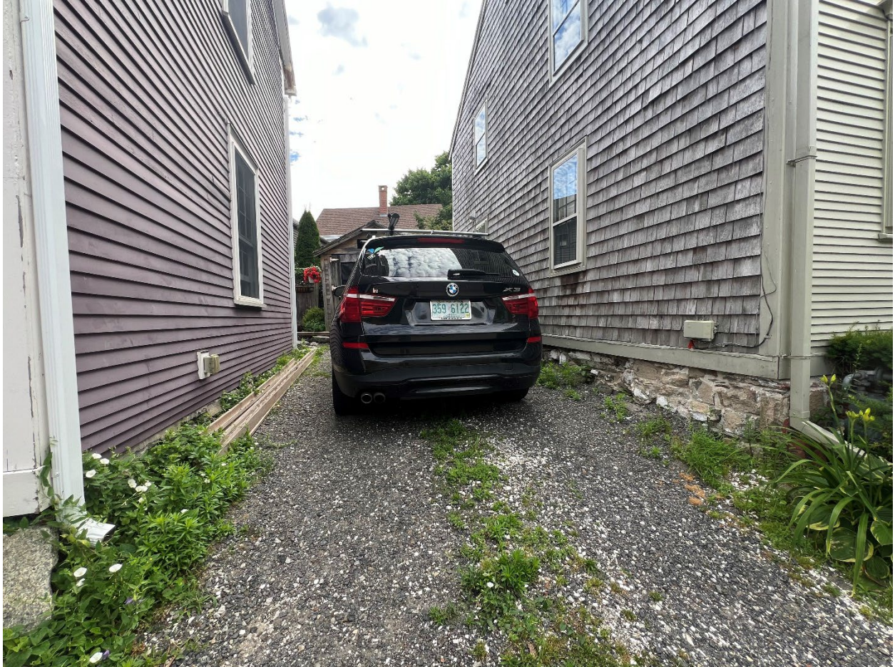
Location of the double arched gate.
