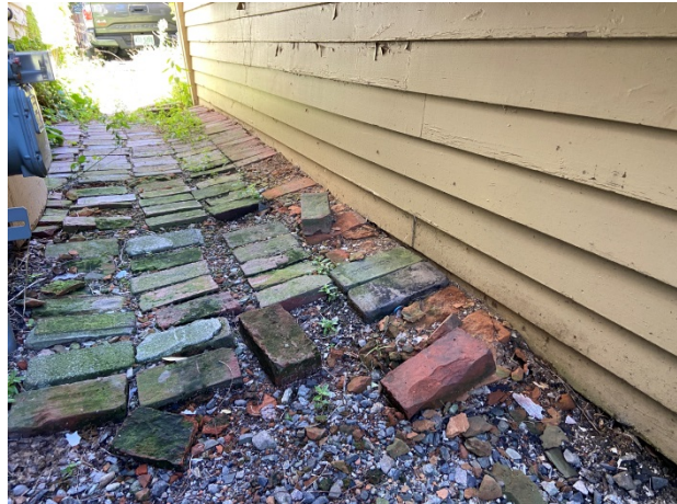
8-Grade along east side
