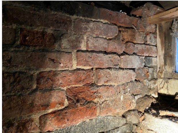
12-Detail of foundation wall
