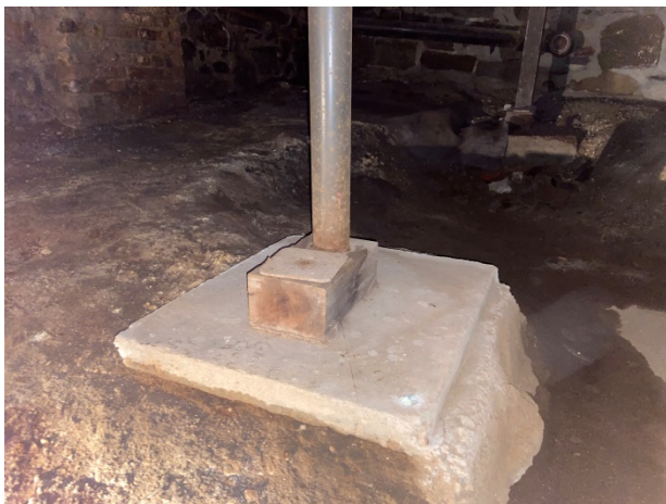
13-Detail of screw jack bearing on wood
