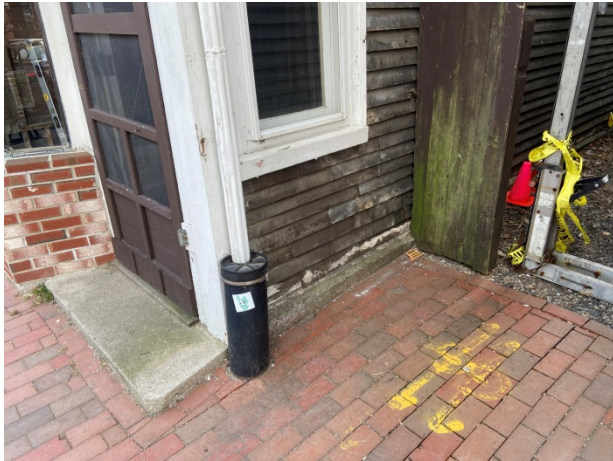
5-Detail at northwest corner
