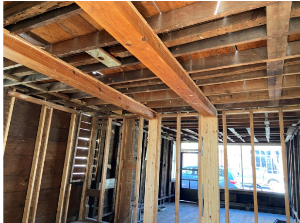
24-Second floor framing
