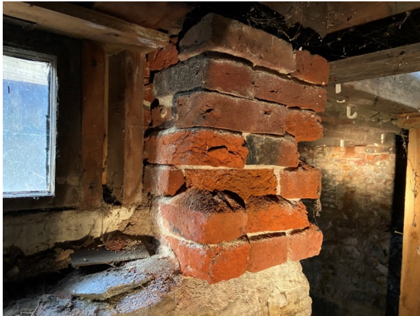
11-Detail of foundation wall
