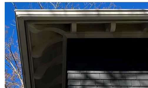
4) ROOF SWEEP AND RAFTER TAILS [FROM BELOW]
