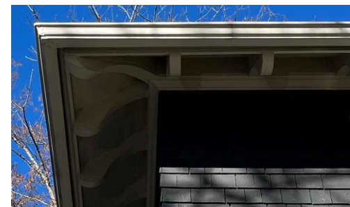
4) ROOF SWEEP AND RAFTER TAILS [FROM BELOW]
