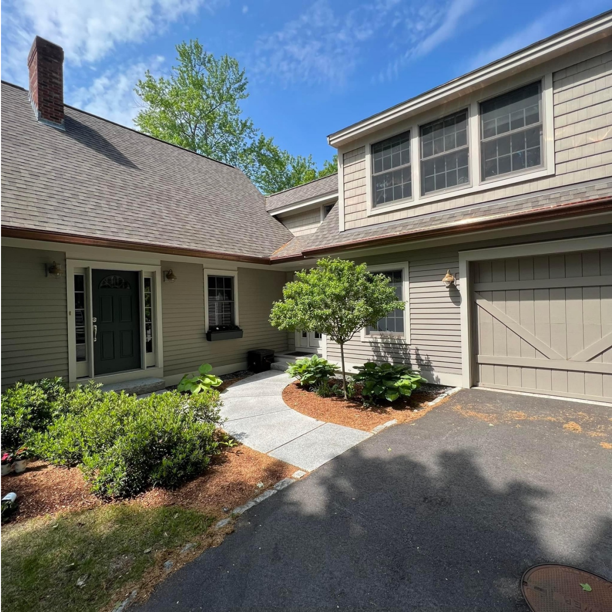
Images of Proposed Gutter installed on Another Home (these images do not show round downspouts, which have been quoted to match existing round downspouts on home)
