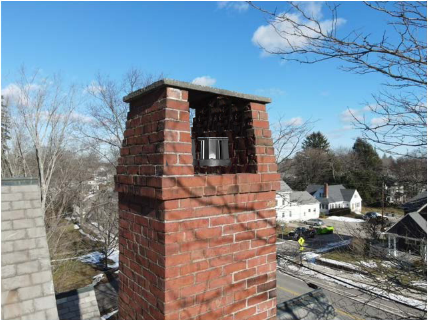
PROPOSED CHIMNEY WITH DIVIDER REMOVED AND TWO TERMINATION CAPS (ONE IS VISIBLE IN THIS IMAGE)
