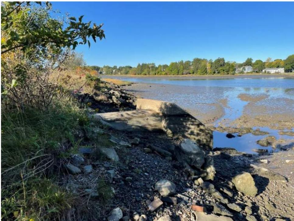
**Photo 4** – Existing outfall headwall, exposed 48” RCP pipe, and tidal embankment looking west at approximate low tide.
