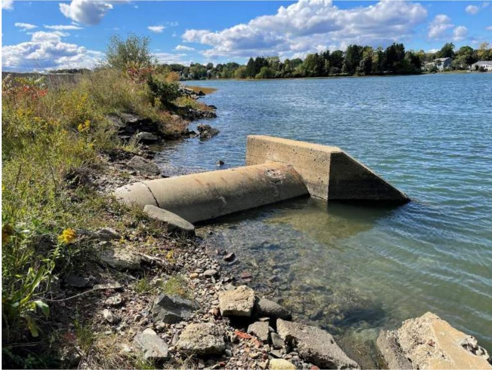
**Photo 1** – Existing outfall headwall, exposed 48” RCP pipe, and tidal embankment looking west at approximate high tide.
