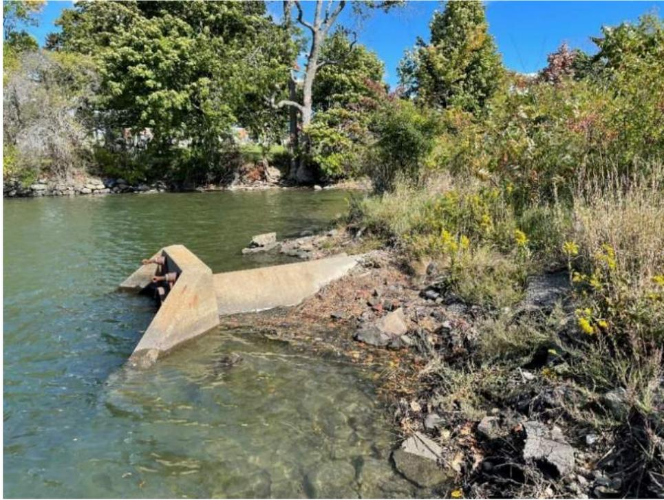
**Photo 3** – Existing outfall headwall, exposed 48” RCP pipe, and tidal embankment looking east at approximate high tide.
