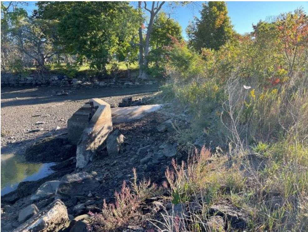
**Photo 6** – Existing outfall headwall, exposed 48” RCP pipe, and tidal embankment looking east at approximate low tide.
