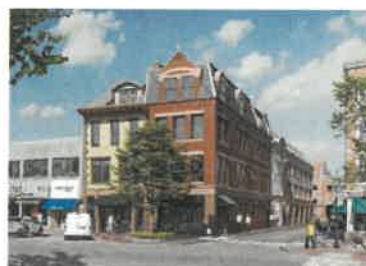
1 Congress Street – Deep energy Retrofit & Addition, Mixed Use – reduce energy usage by 70% beyond baseline 20
