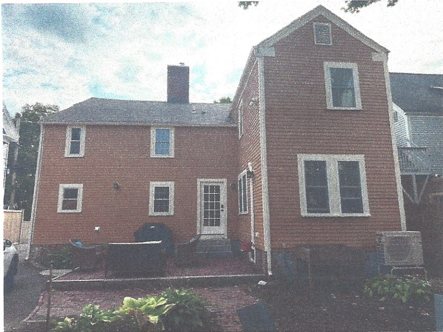
1. View of the back of the existing house at 47 Langdon Street
