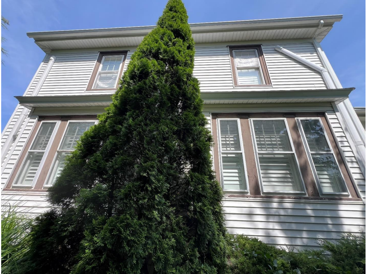
Left side view of House at 271 Sagamore Avenue
