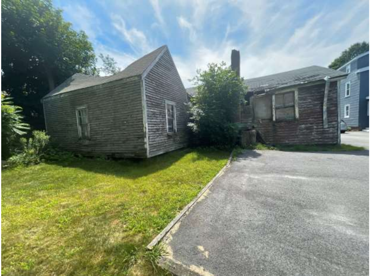
Accessory Building (Rear View)
