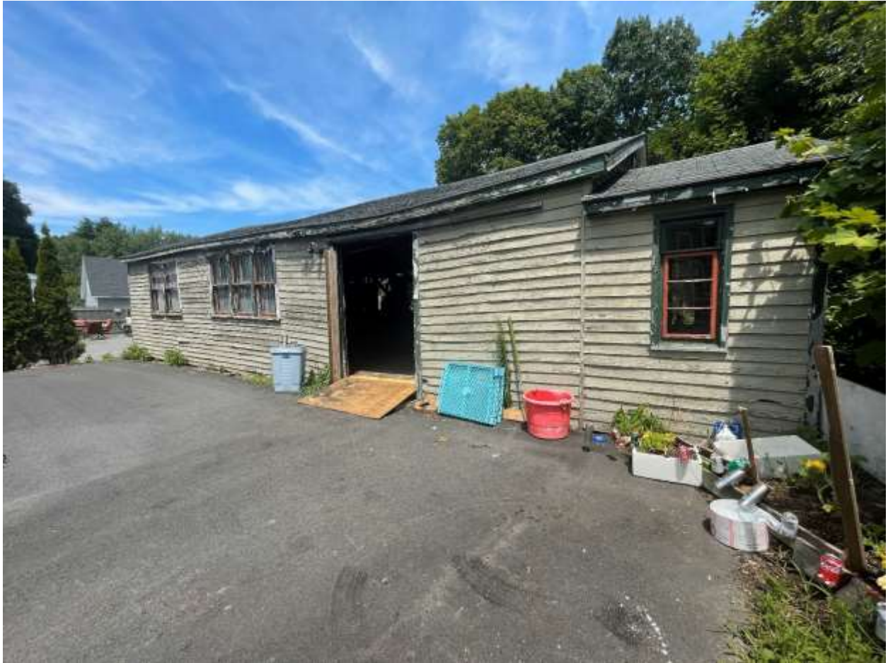
Accessory Building (Front View)
