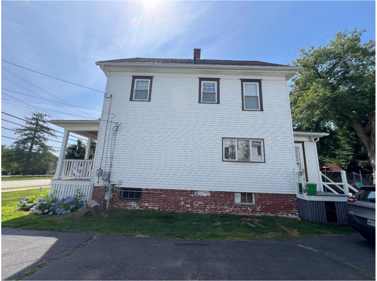
Right side view of House at 271 Sagamore Avenue
