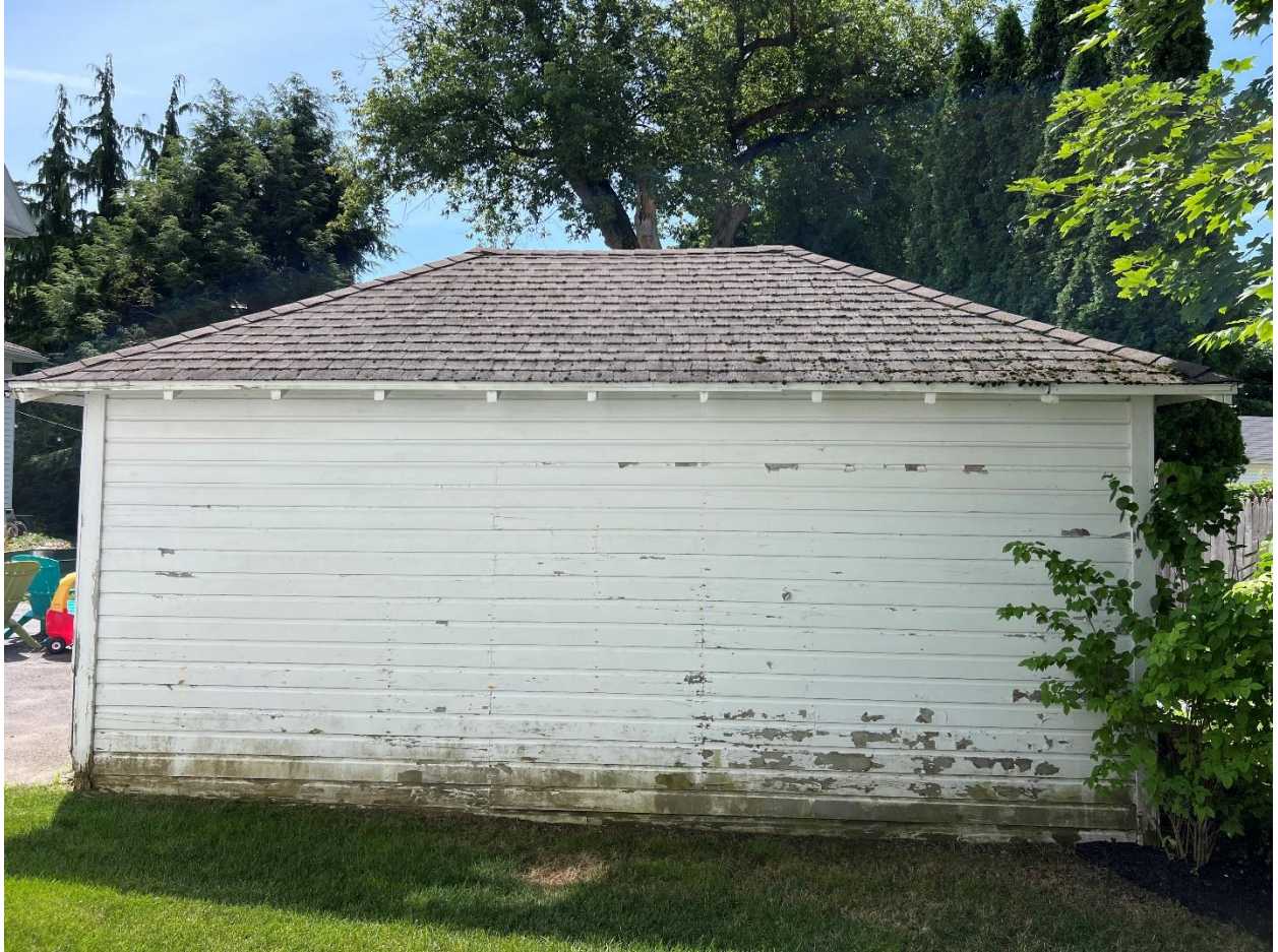
Right side view of Garage at 271 Sagamore Avenue
