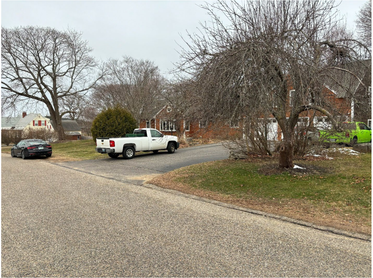
Front View from Farm Lane (South Elevation View)
