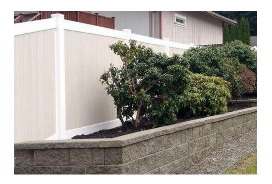
These are three images of the currently constructed/installed retaining wall, which is approximately 38 inches – 40 inches above soil. The frequent and intense weather conditions, including rainfall and recent snow, have caused the final calculation of the retaining wall above ground to fluctuate. But the final result is planned to be 38 inches of retaining wall above ground with plantings in front of the fence and the wall.
