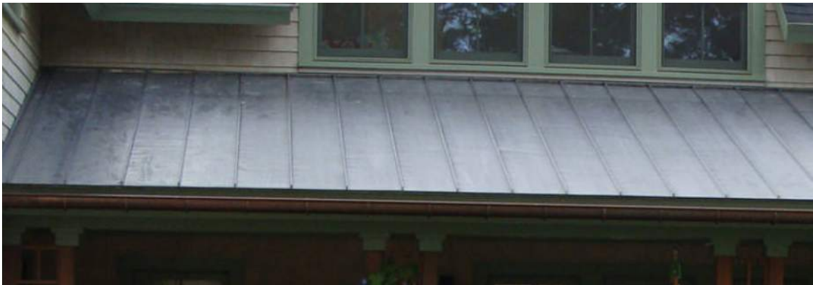
STANDING SEAM LEAD COATED COPPER ROOF
