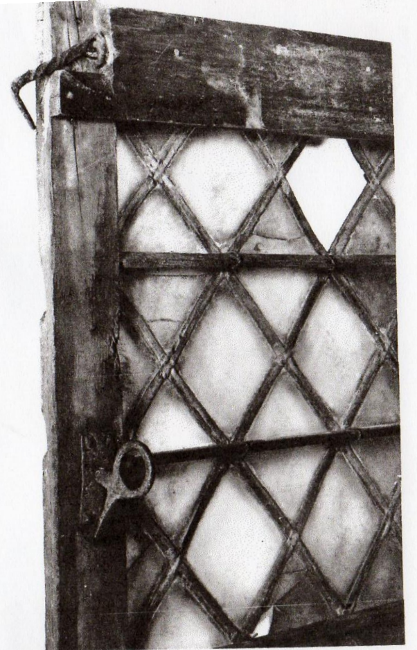
Figure 200B. Buffum house, Salem, Mass., probably seventeenth century. Demolished. Casement window sash, detail of interior surface (with later board reinforcement along upper rail). Photo, J. David Bohl, 1978.
