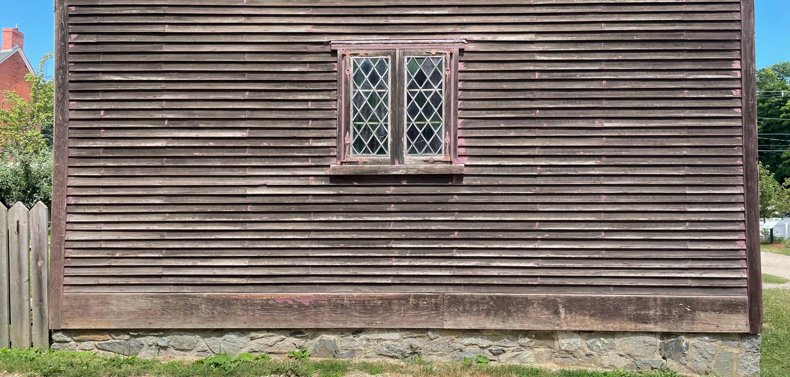
Existing West Window
