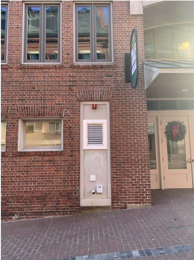
LOUVER FROM CHESTNUT STREET LOCATED IN EXISTING PANELING WITH OTHER MECHANICAL PENETRATIONS
