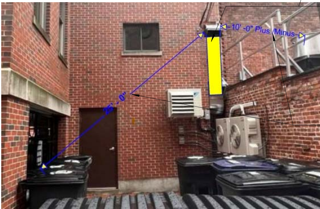
EXISTING GOOSENECK INTAKE GRILL IS NOT IN MECHANICAL CODE COMPLIANCE: WITHIN 10'-0" OF EXHAUST FAN AND 25'-0" OF POTENTIAL CAR EXHAUST
