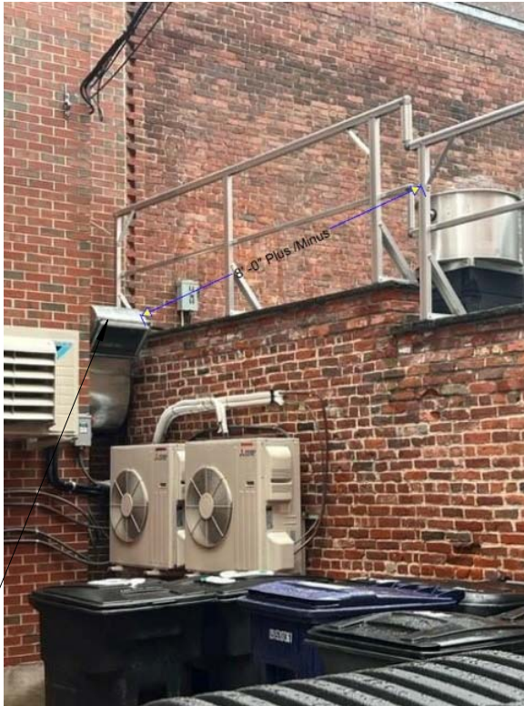
EXISTING GOOSENECK INTAKE GRILL IS NOT IN MECHANICAL CODE COMPLIANCE: WITHIN 10'-0" OF EXHAUST FAN AND 25'-0" OF POTENTIAL CAR EXHAUST
