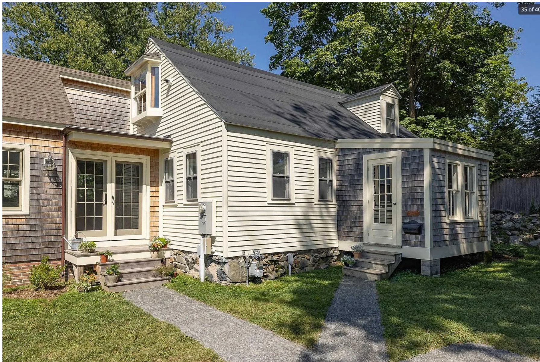
EXISTING VIEW OF ENTRY AND MUDROOM AREA
