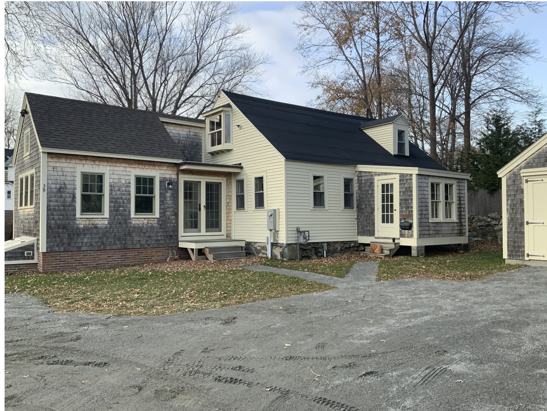
EXISTING FRONT HOUSE
