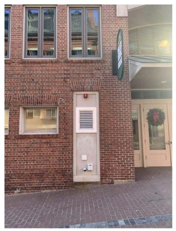
LOUVER FROM CHESTNUT STREET LOCATED IN EXISTING PANELING WITH OTHER MECHANICAL PENETRATIONS
