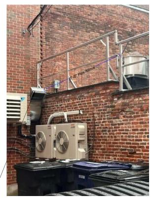
EXISTING GOOSENECK INTAKE GRILL IS NOT IN MECHANICAL CODE COMPLIANCE: WITHIN 10'-0" OF EXHAUST FAN AND 25'-0" OF POTENTIAL CAR EXHAUST
