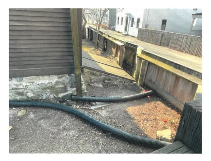
Would like to remove these drainpipes and excavate a new underground drainage pipe with crushed stone and rubber membrane under the surface.
