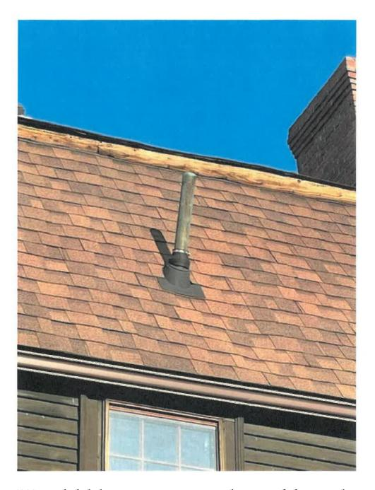
Would like to remove this rubber plumbing roof vent with custom lead coated copper vents.
