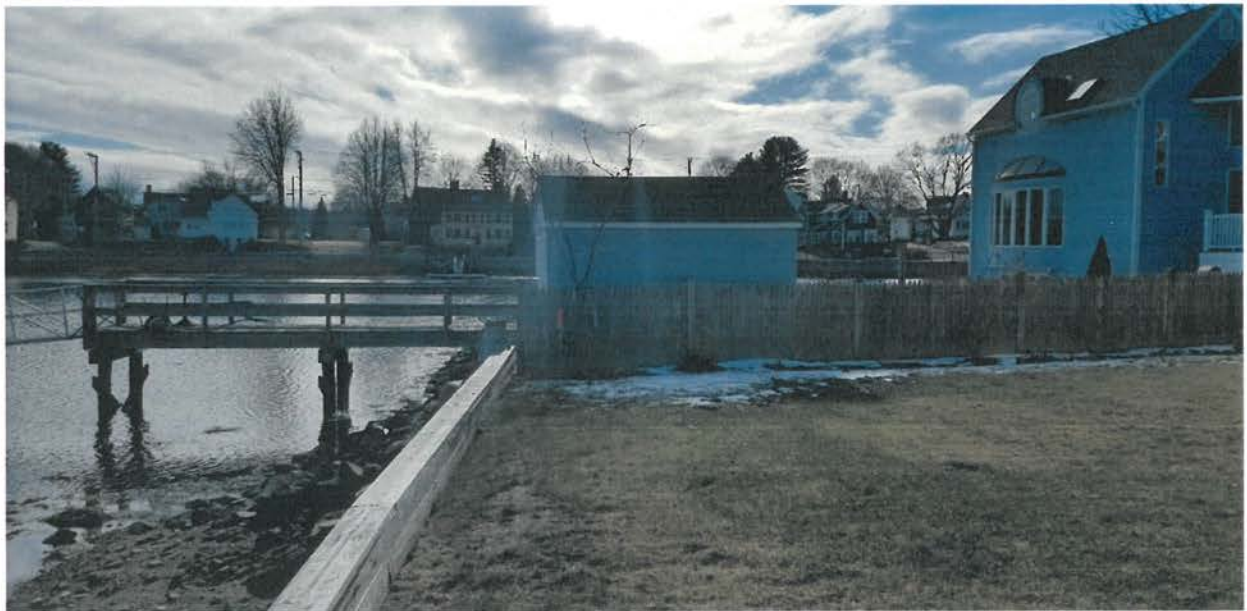
Photo 11 – Looking southerly in the backyard along the retaining wall - January 11, 2023.
