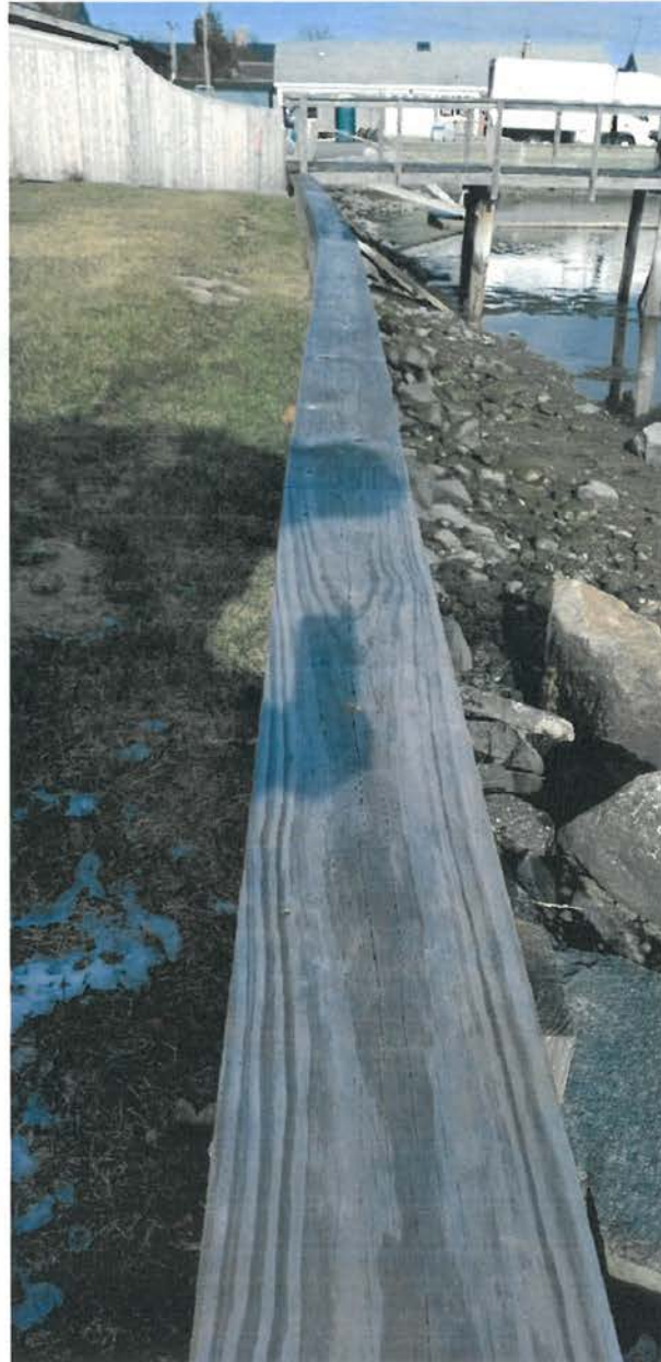
Photo 7 – Looking northerly along the retaining wall in the backyard - January 11, 2023.
