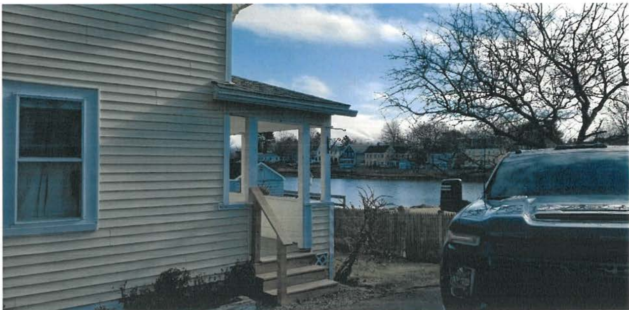
Photo 4 – Looking easterly at the water and 43 Holmes Court - January 11, 2023
