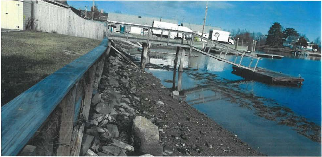
Photo 8 – Looking northerly along the retaining wall along the Piscataqua River - January 11, 2023.
