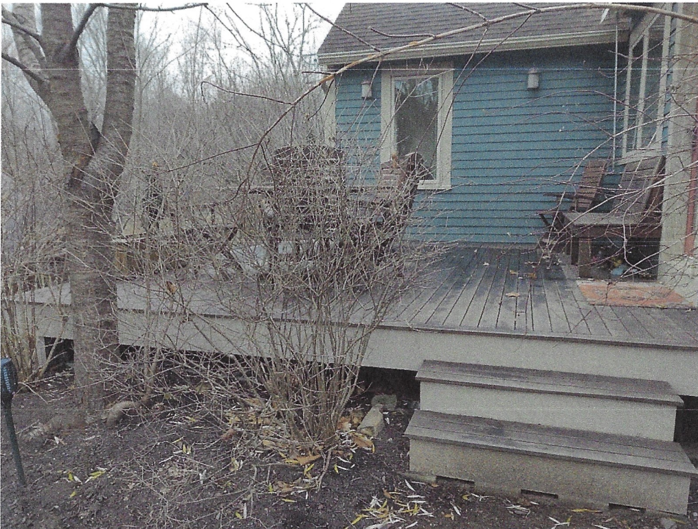
4. A close up of the deck where the addition is proposed.
