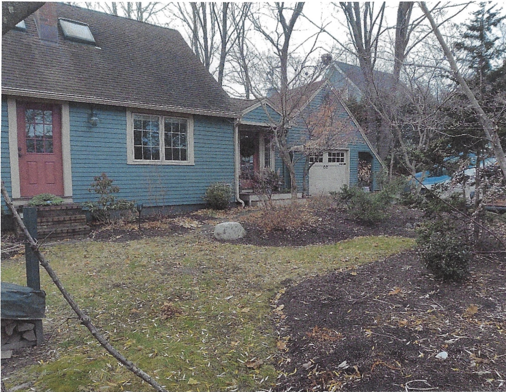
5. Looking west at the front door where the new entrance is proposed and new landscaping.
