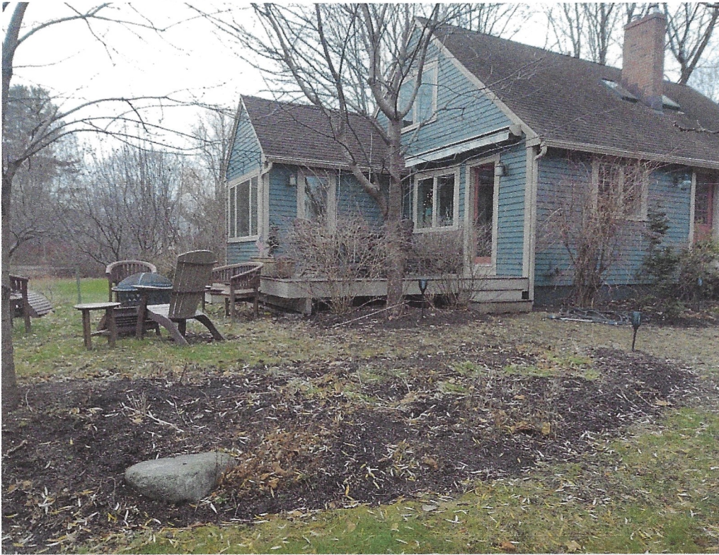
3. Looking west at the deck where the addition is proposed. The temporary impacts will start on the far side of the landscape bed in the foreground.
