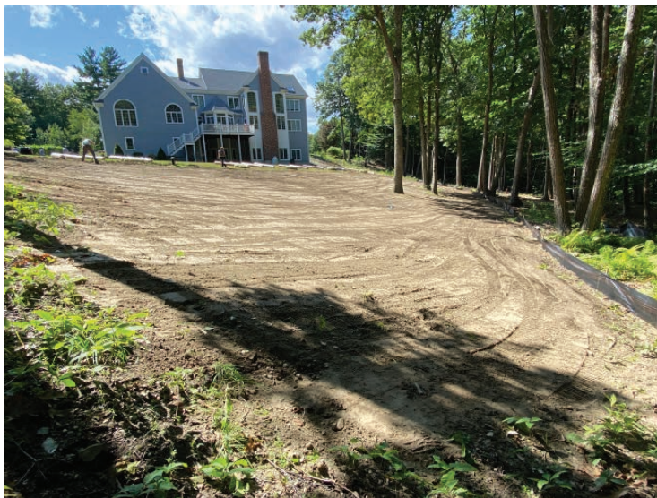
2. After installation of sediment control, we mechanically mowed area and seeded with New England Conservation and Wildlife Seed Mix
