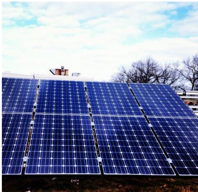
Completed installation showing gaps between panels
