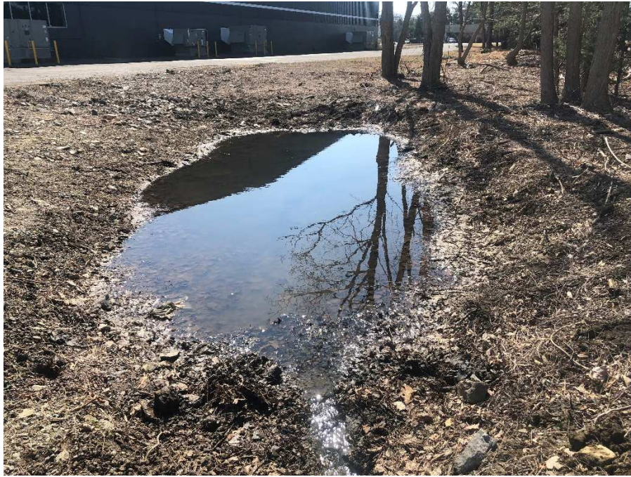
View of existing stormwater pond
