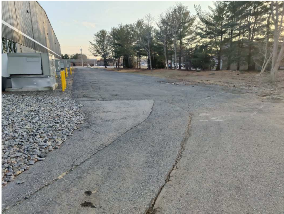
View of building & parking lot looking to the south
