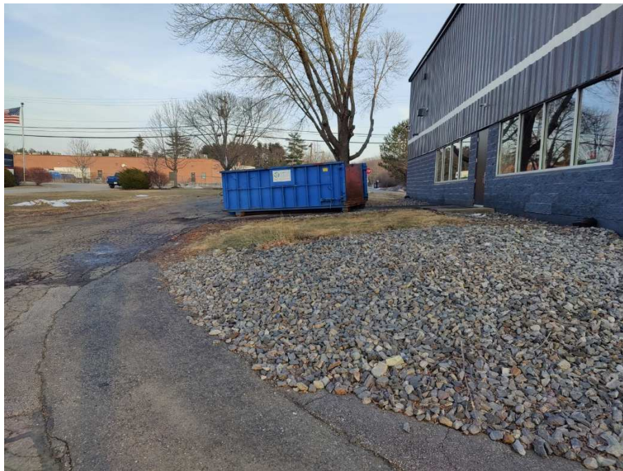
View of building looking to the east
