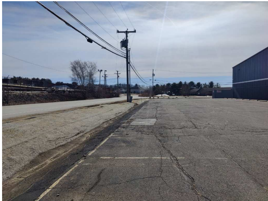
View of front parking lot & swale looking to the south
