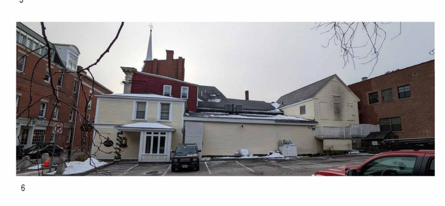
H2.04 EXISTING CONDITIONS PHOTOS 1 CONGRESS STREET SCALE: 8000000
