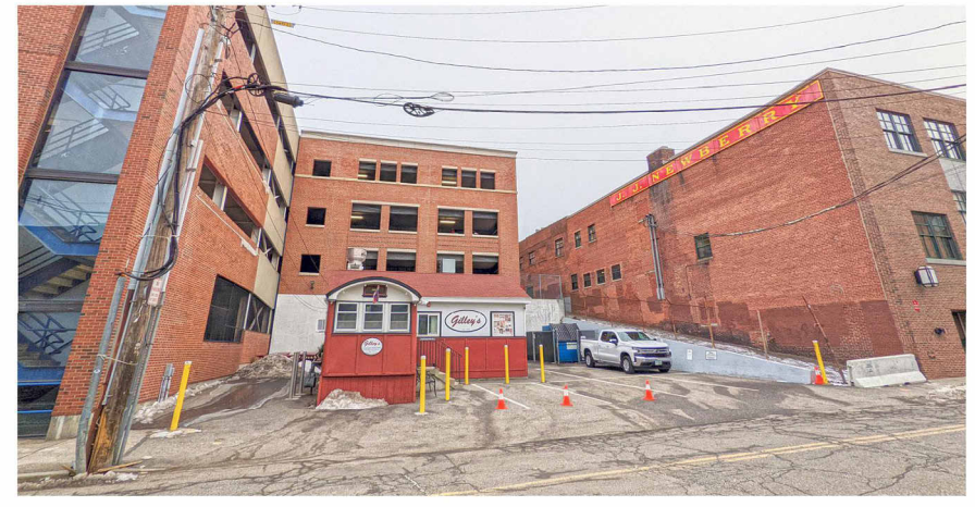
HAVEN COURT AT FLEET STREET
