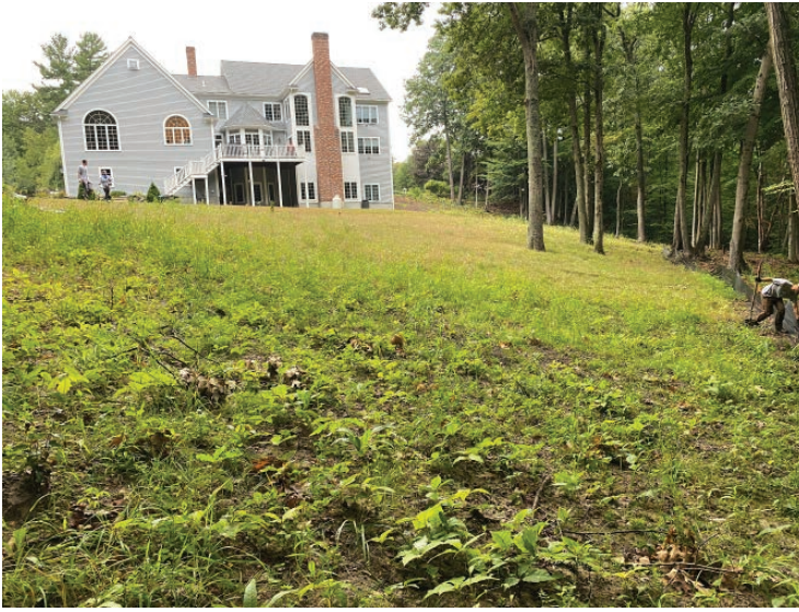
1. Existing Conditions - Client under an enforcement order to restore buffer after tree & shrub removal and hydroseeding turf
