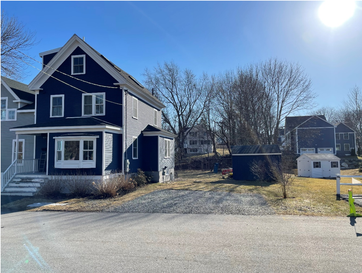
Front View (from Monteith St)
